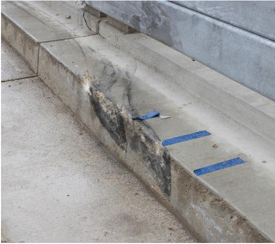
(a) Traffic side at impact point
