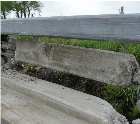
(a) Section 3 just downstream of joint 2
