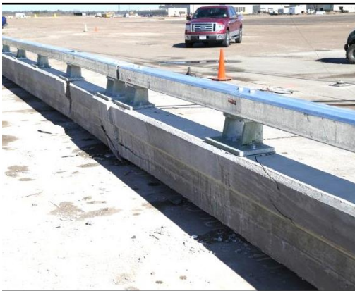
(c) Field side of bridge rail
