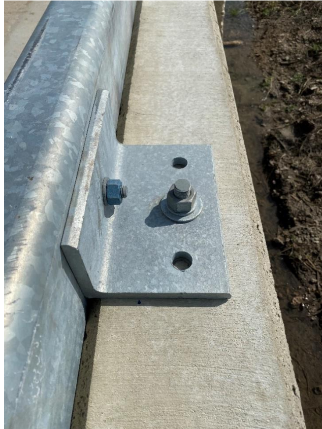
Figure 94. Installed L6×4×½ angle support bracket with ¾-in. A193 B7 galvanized threaded rod with Hilti RE500-V3 adhesive
