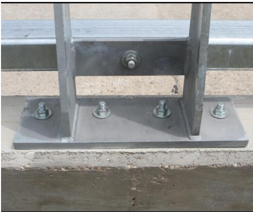
(e) Field side of post connection
