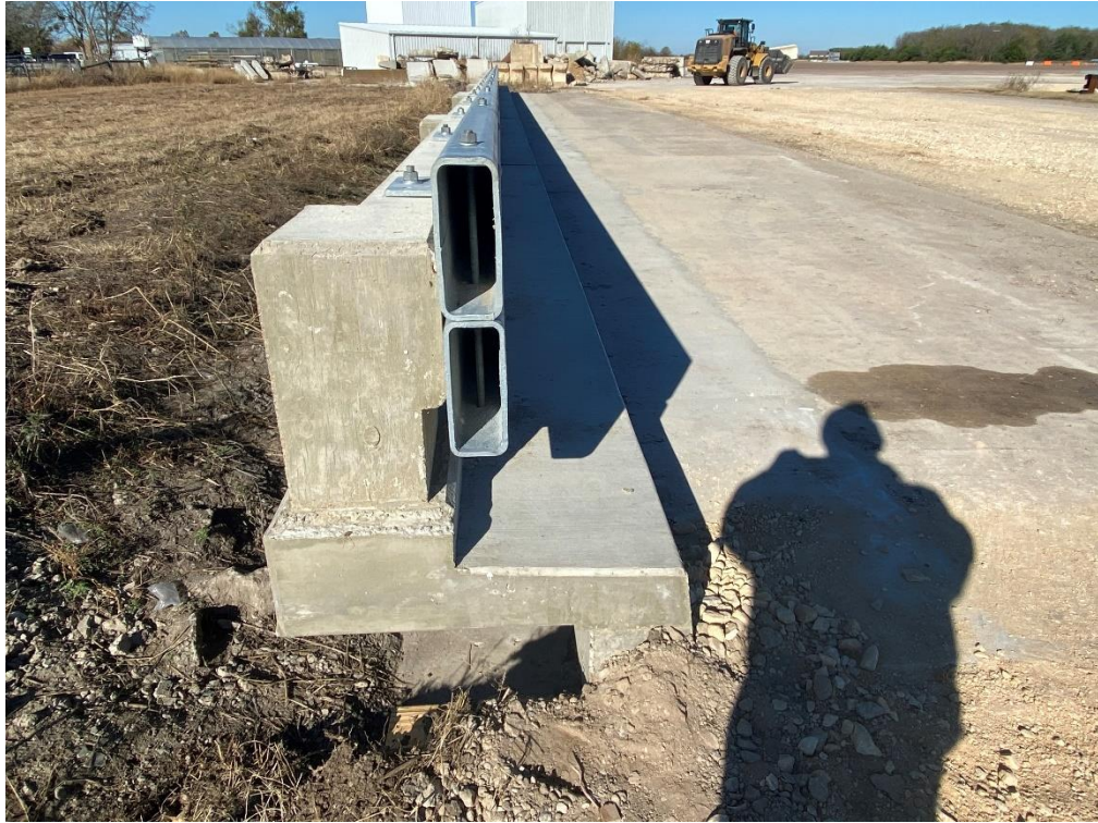
Figure 99. End view completed retrofit rail installation
