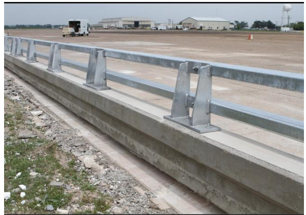
(f) Field side of bridge rail
