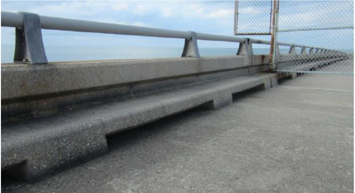
Figure 1. Photo of the old southbound causeway bridge rail
