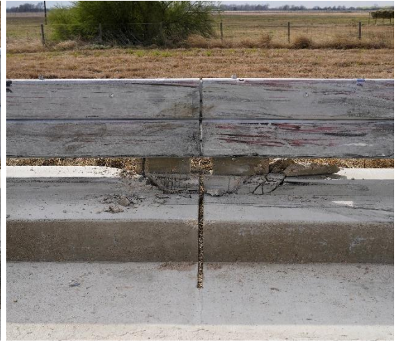
(b) Traffic side of joint
