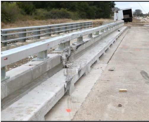
(a) Traffic face of bridge rail
