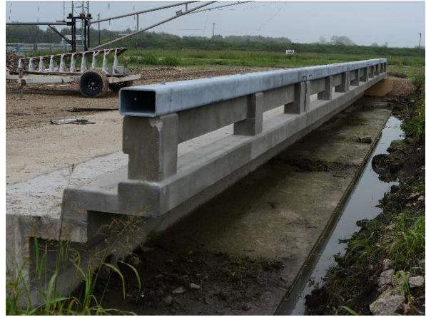
(b) Field side of bridge rail
