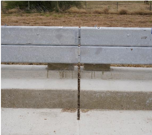
(a) Traffic face at joint
