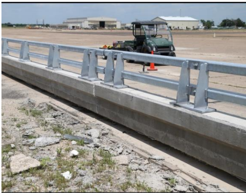
(c) Field side of bridge rail
