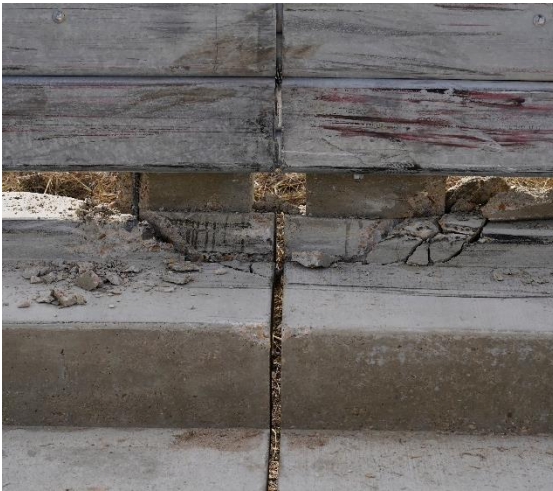
(c) Traffic side of posts at joint
