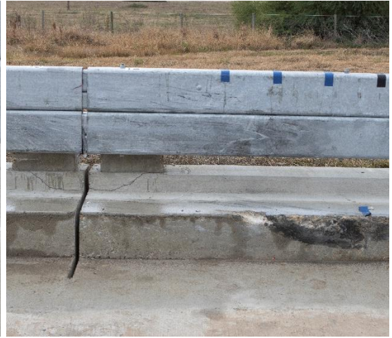
(b) Traffic side of joint
