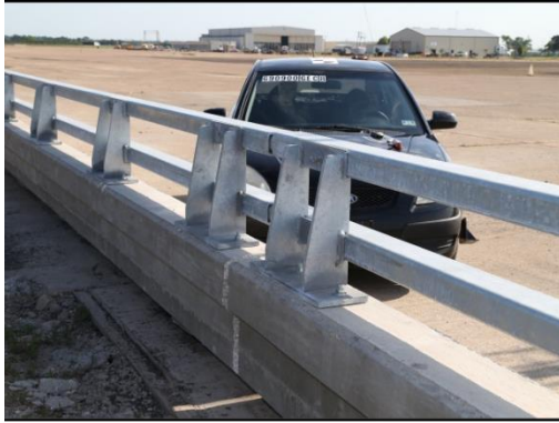
(a) 1100C test vehicle and bridge rail
