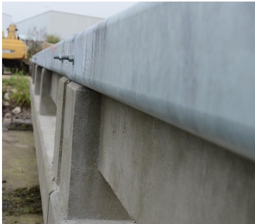
(a) Field side of joint 2
