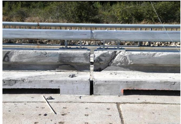
(b) Traffic side of joint
