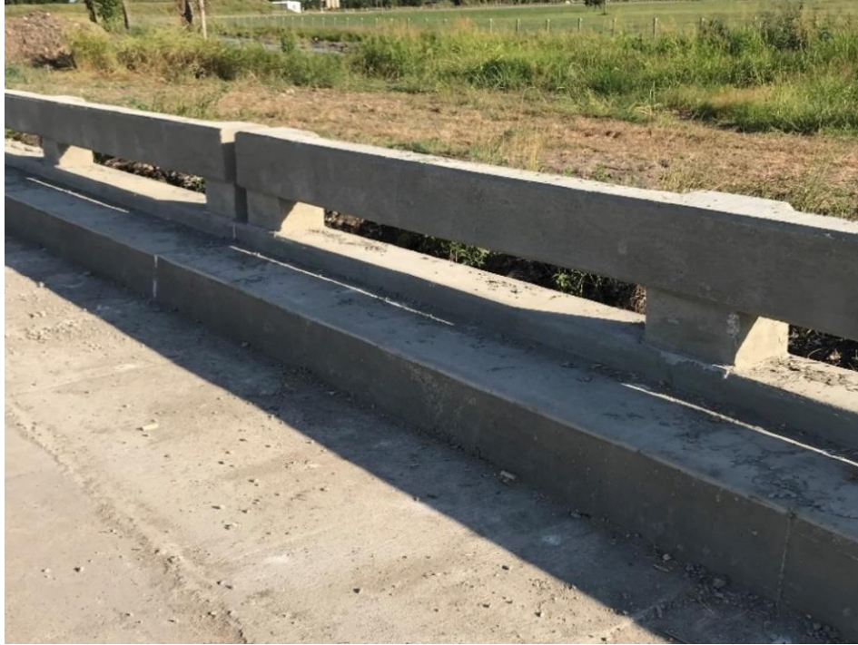
Figure 91. Safety walk barrier with concrete post and beam bridge rail
