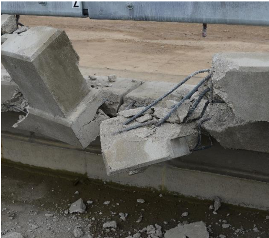
(c) Field side of end posts at joint 2
