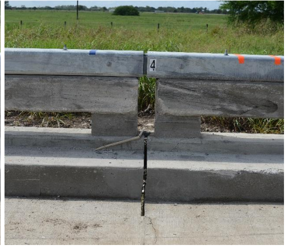
(b) Traffic side of joint 4
