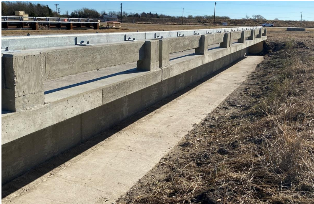
Figure 100. Field side view completed retrofit rail installation
