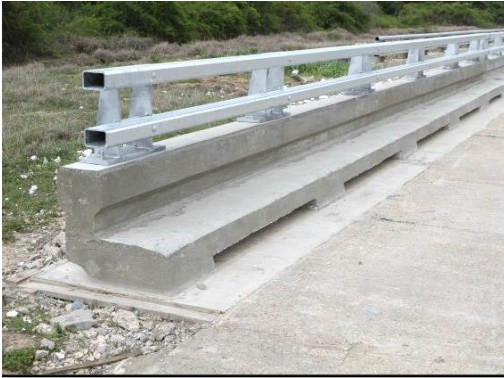
(a) Traffic face of bridge rail
