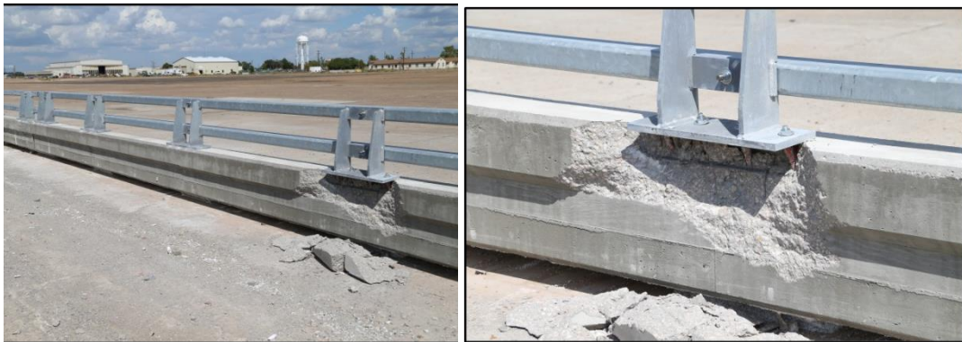
(b) Damage at post 9
