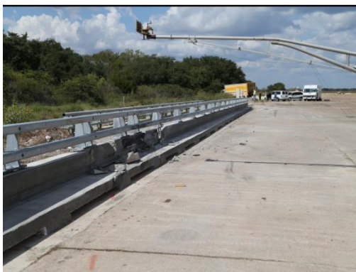
(a) Traffic side of bridge rail
