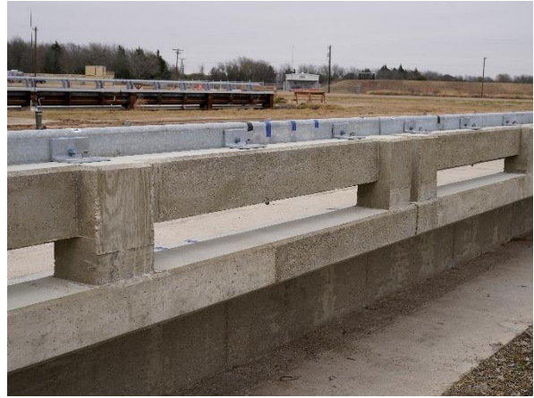
(b) Field side of bridge rail
