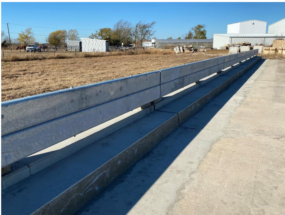
Figure 98. Front view completed retrofit rail installation
