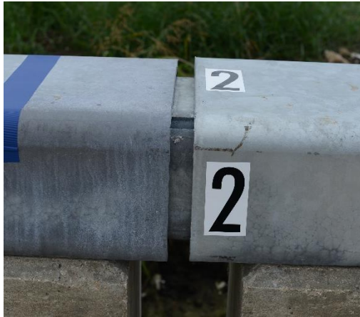
(a) Metal rail element at joint 2
