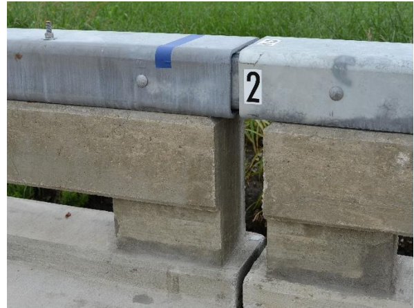
(b) Concrete parapet at joint 2
