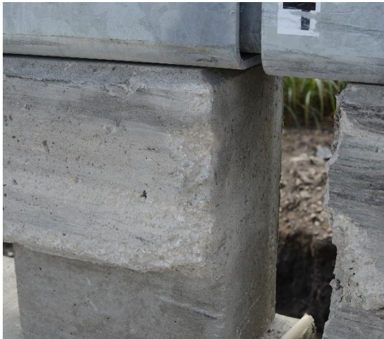
(c) Traffic side of posts at joint 4
