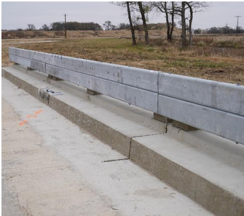
(c) Upstream of joint
