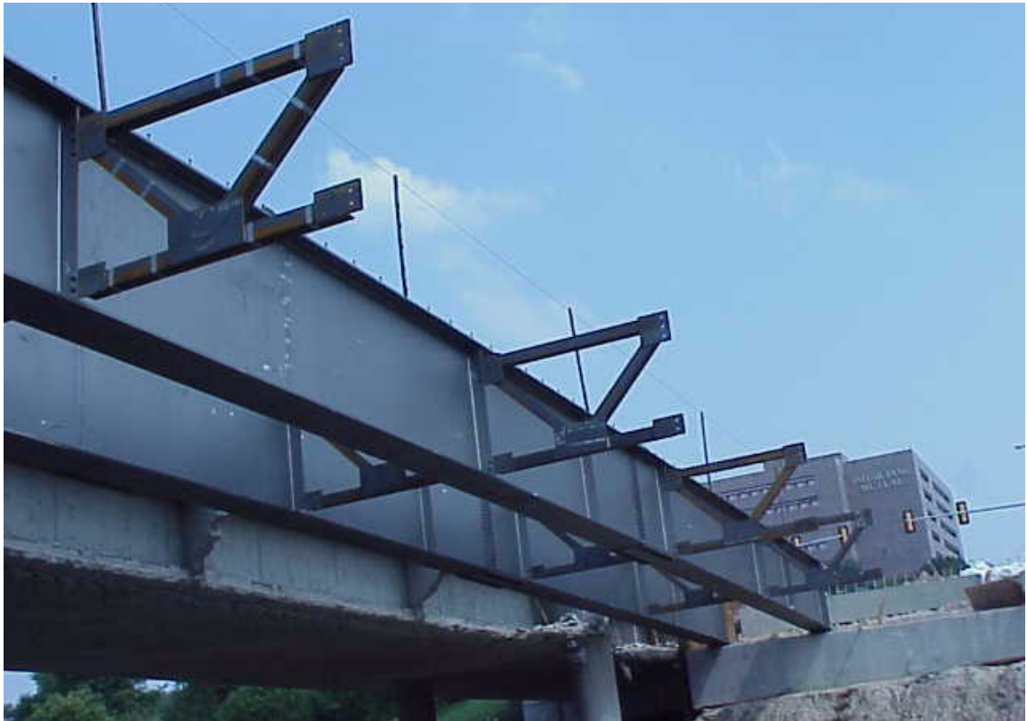
Figure 2-11: Girder sections 4 and 5 of the East span
