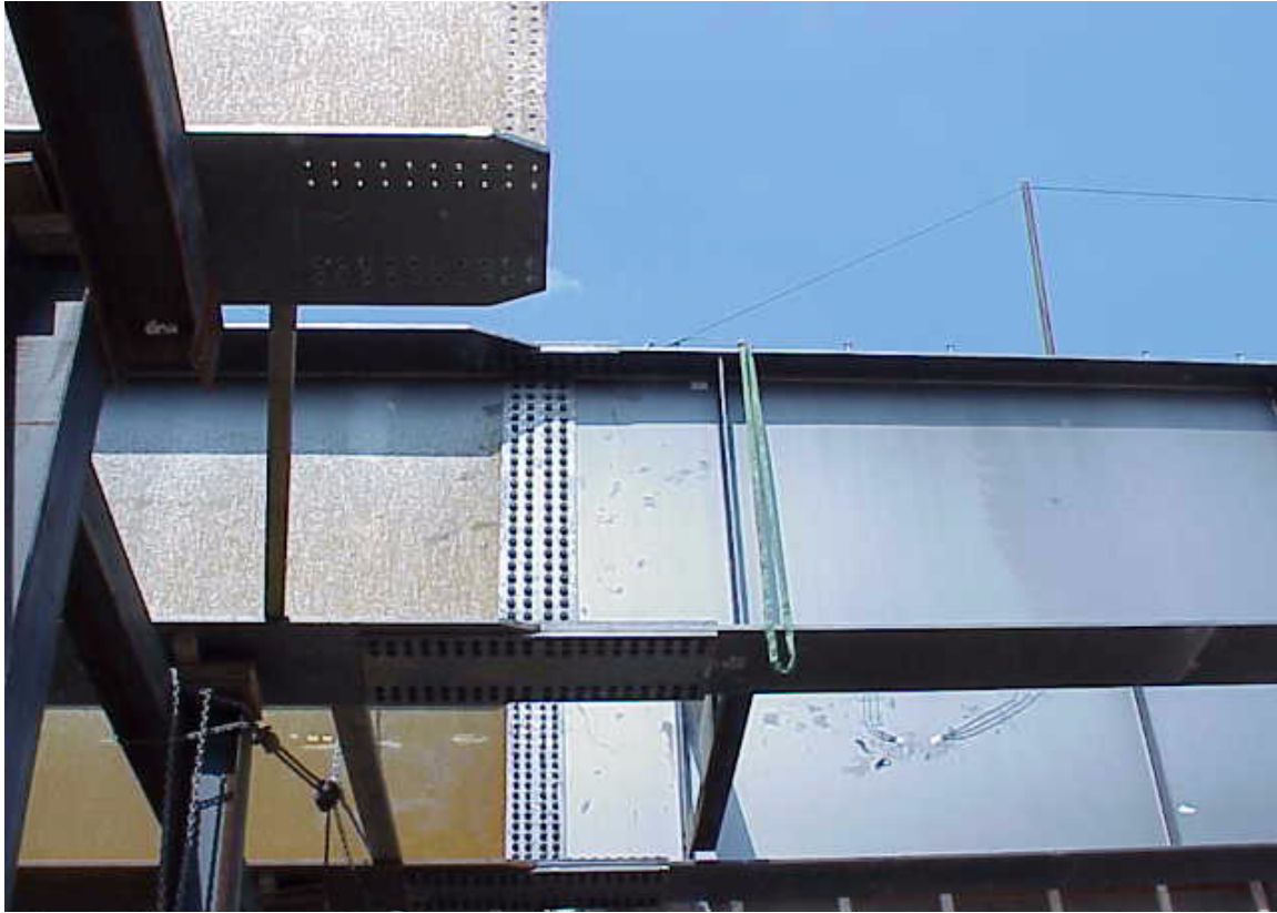
Figure 2-14: Girder splice
