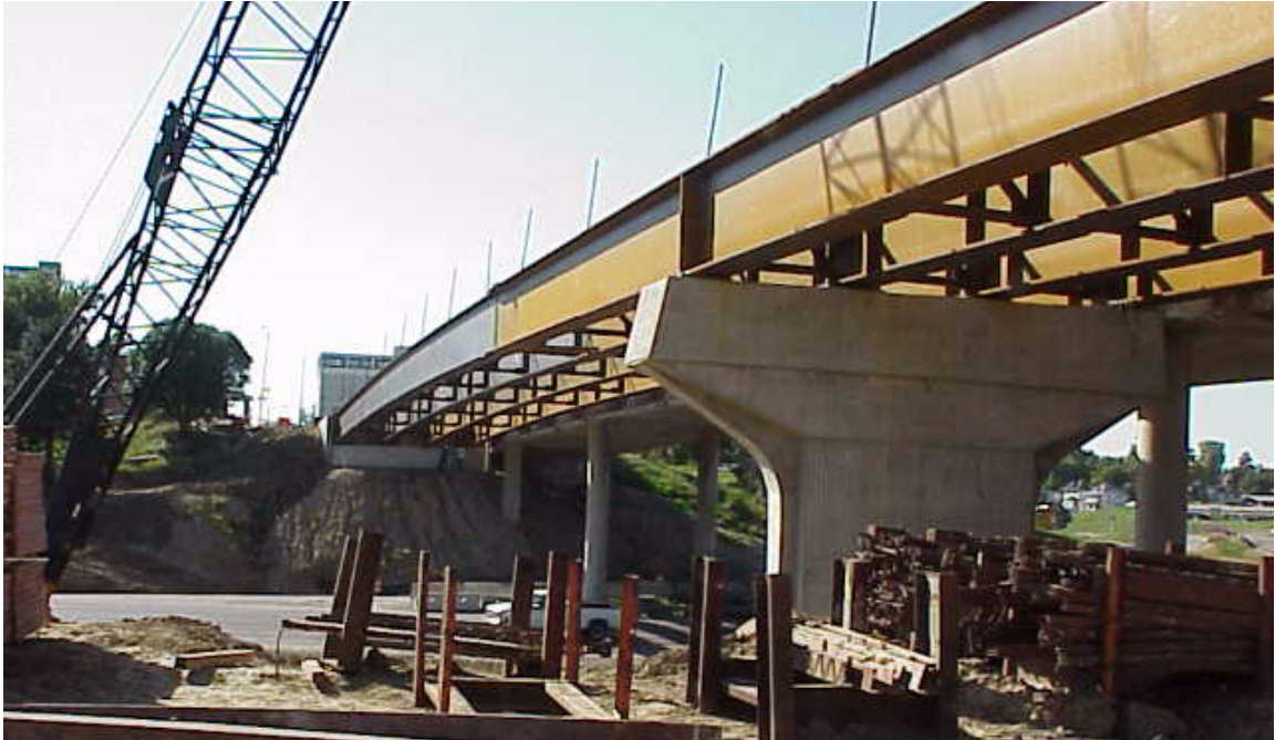
Figure 2-13: West span girders in place
