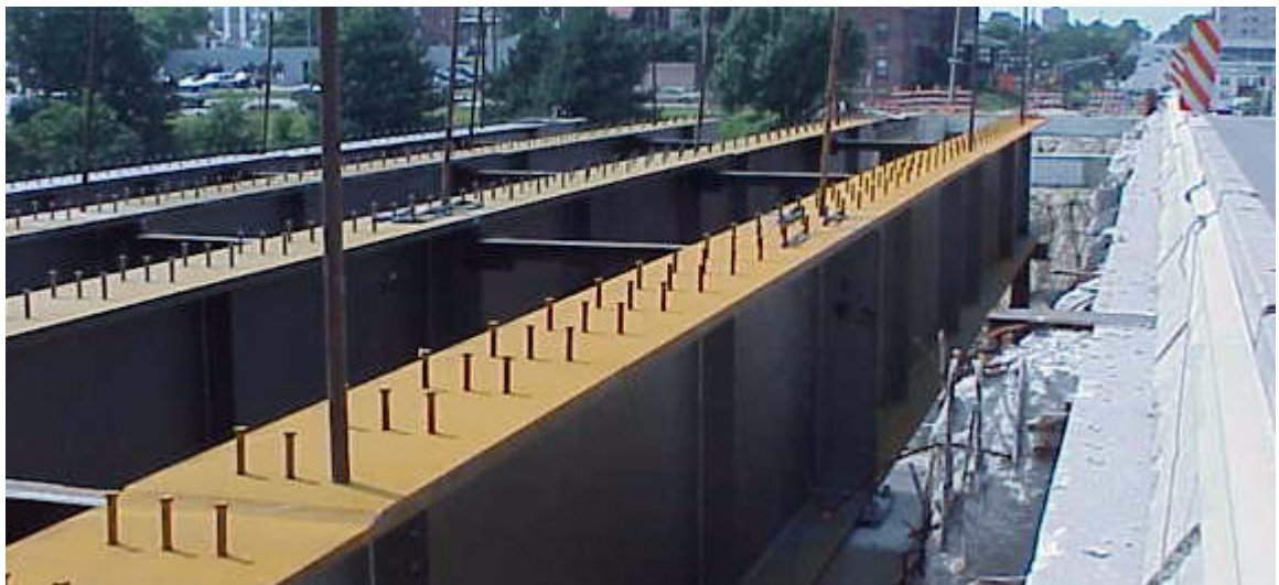
Figure 2-4: Shear Studs on the top flange. Picture is taken looking West. From right to left are Girders E, G, H, and J during erection for Phase I.
