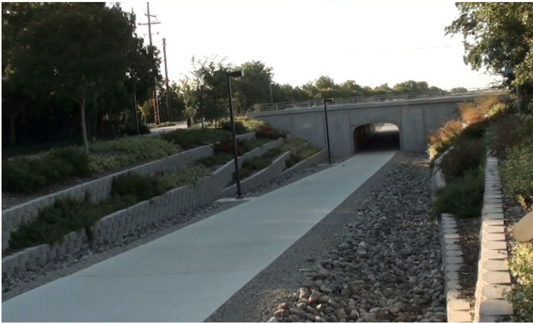
Figure 47. Underpass for Bicycle Path #2 – Davis, California
