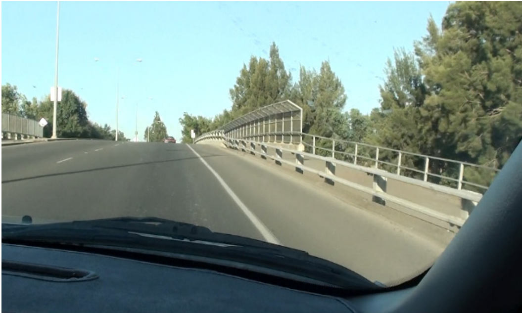
Figure 48. Bicycle Lane on Highway Bridge – Davis, California
