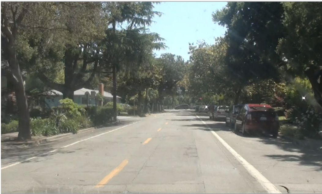
Figure 22. Shared Shoulder for Parking and Bicycling – Palo Alto, California
