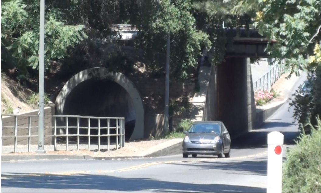
Figure 45. Bicycle Underpass – Davis, California
