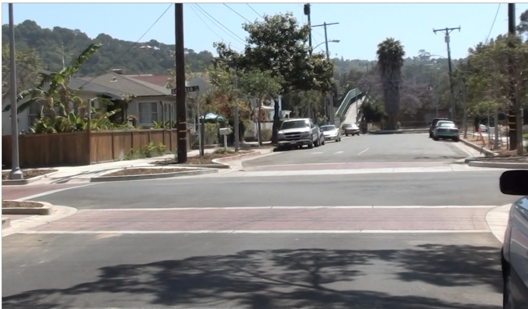
Figure 38. Bulb-out at Intersection to Shorten Crossing – Santa Barbara, California
