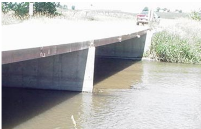
Figure 3 Low water bridge in Benton County, Iowa.
