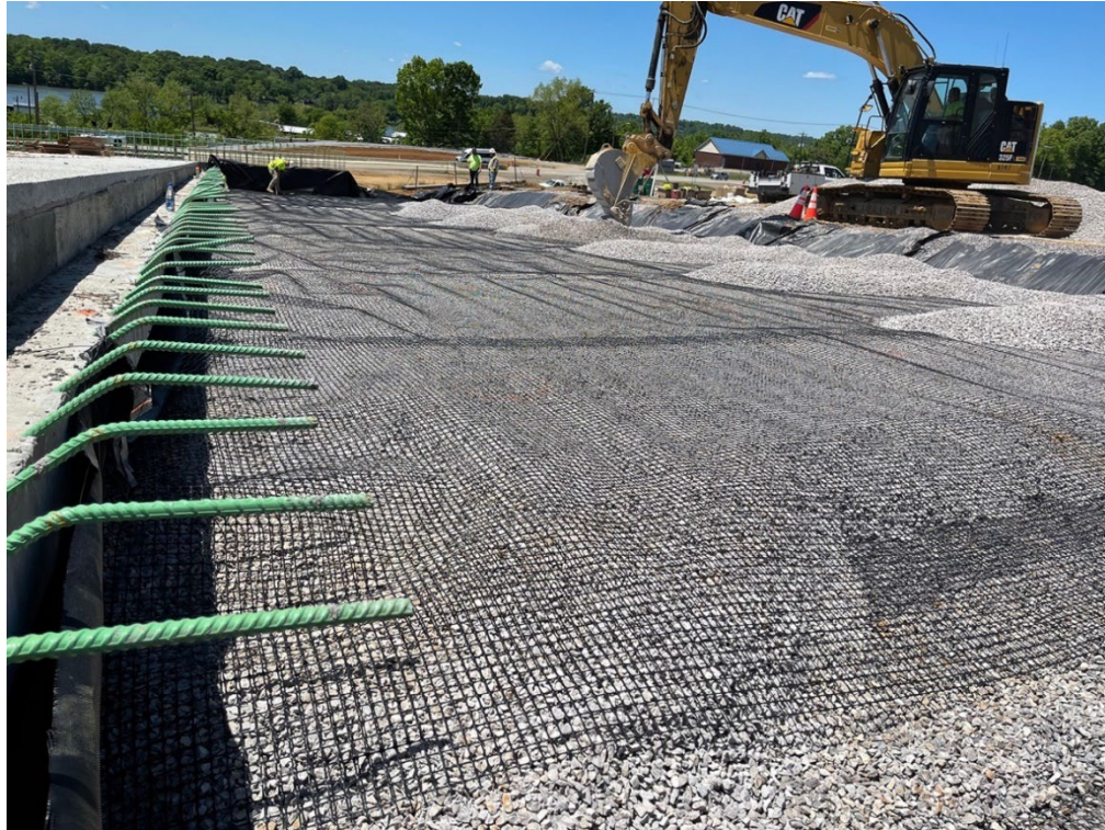
Figure 3-4. Tensar Biaxial BX1200 geogrid placed over #57 stone 9-in. fill.
