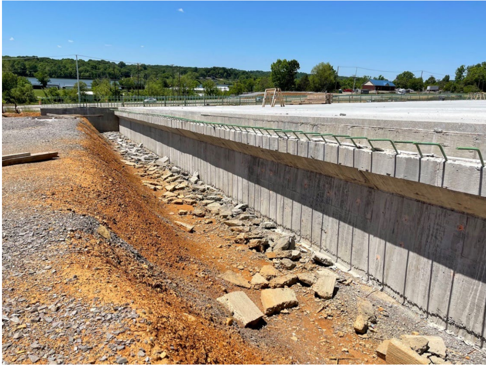
Figure 3-2. Photo of the face of the south abutment before constructing the approach slab.
