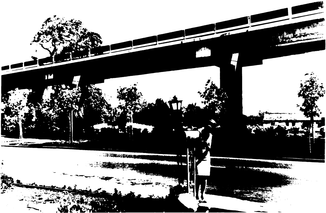
BART's elevated structures created controversy in Berkeley and other parts of the Bay Area
