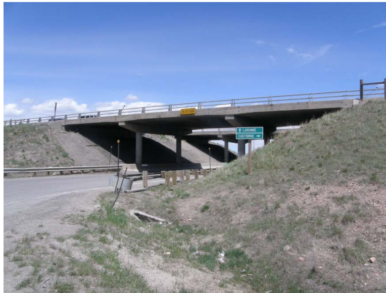
Figure 15: Eastbound Remount Bridge (structure AYB), near Buford, Wyoming.
