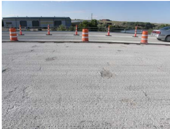
Figure 35: Casper Bridge milled surface (140 ft to 160 ft).
