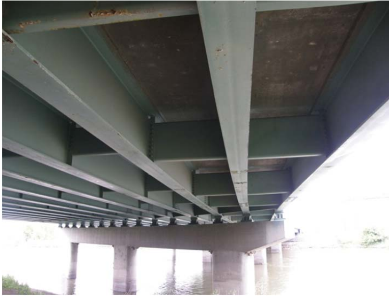
Figure 12: First Street Bridge underside in Casper, Wyoming.
