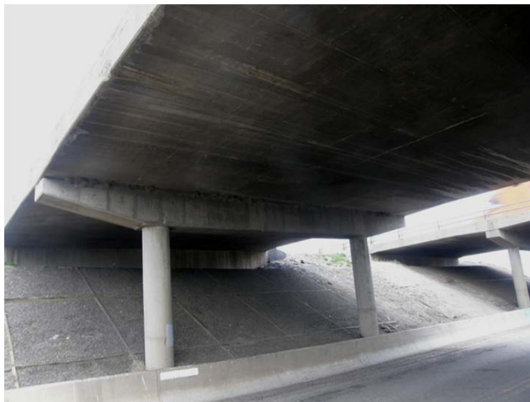
Figure 16: Eastbound Remount Bridge (structure AYB) underside, near Buford, Wyoming.
