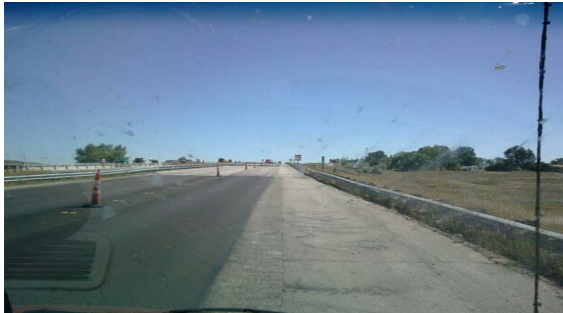
Photograph 1. Bridge on I-25 in Douglas, Converse County,
