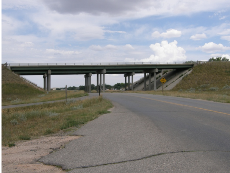
Figure 13: Southbound I-25 (Structure AFY) Bridge in Douglas, Wyoming.
