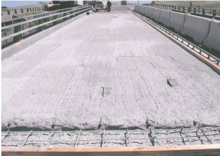
Figure 54: Remount Bridge reconstruction.
