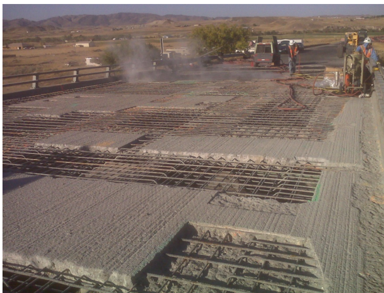
Figure 45: Douglas Bridge chipping looking east.
