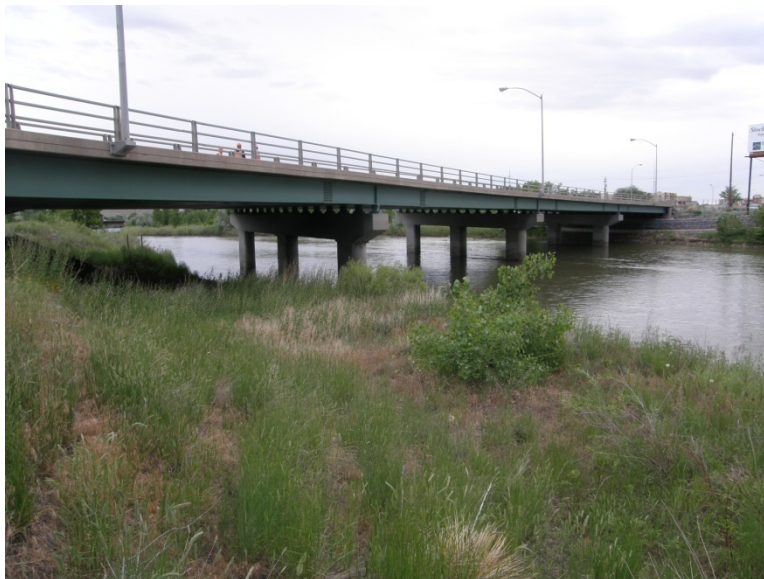
Figure 11: First Street Bridge in Casper, Wyoming.
