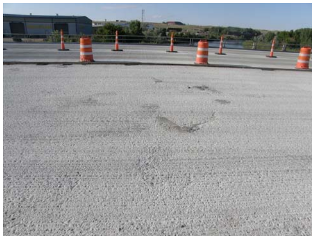
Figure 36: Casper Bridge milled surface (160 ft to 180 ft).
