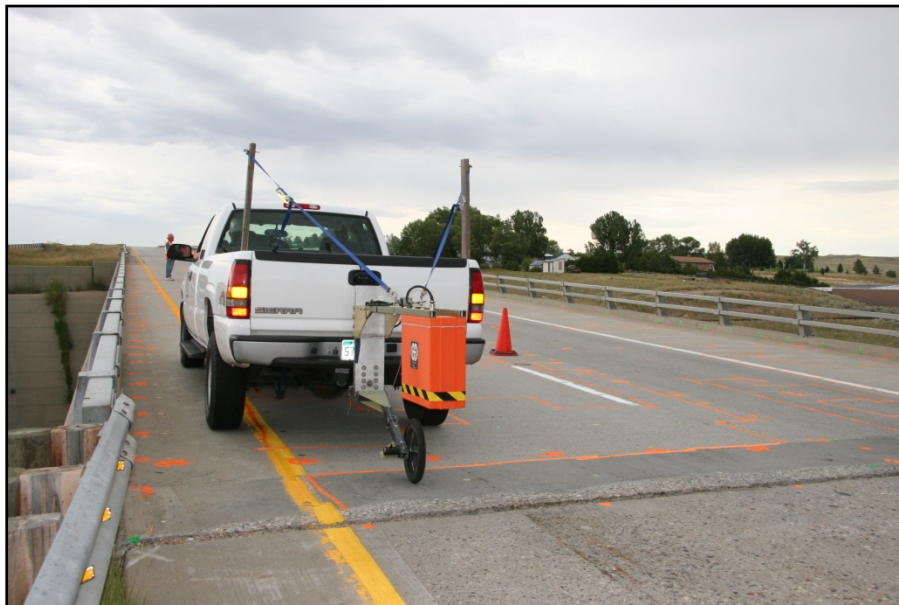
Figure 3 - GPR testing with the 2GHz air horn antenna on I-25 in Douglas Wyoming.
