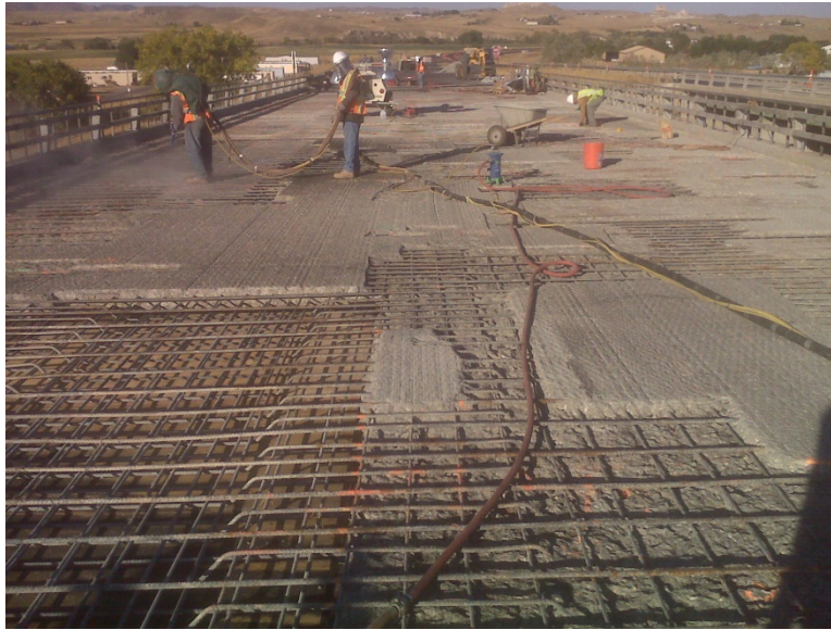
Figure 44: Douglas Bridge chipping looking east.
