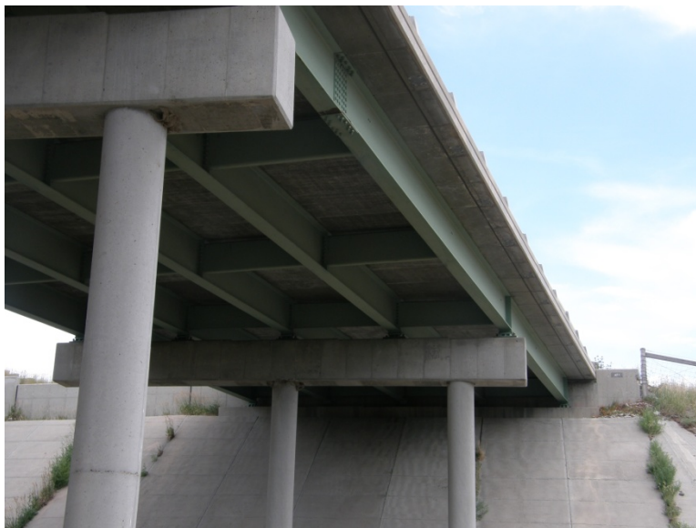
Figure 14: Southbound I-25 (Structure AFY) Bridge underside in Douglas, Wyoming.
