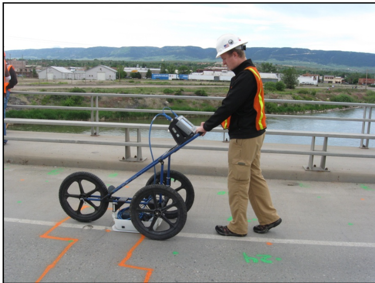
Figure 3 - GPR testing with the 1500MHz ground-coupled antenna over the North Platte River in Casper, Wyoming.
