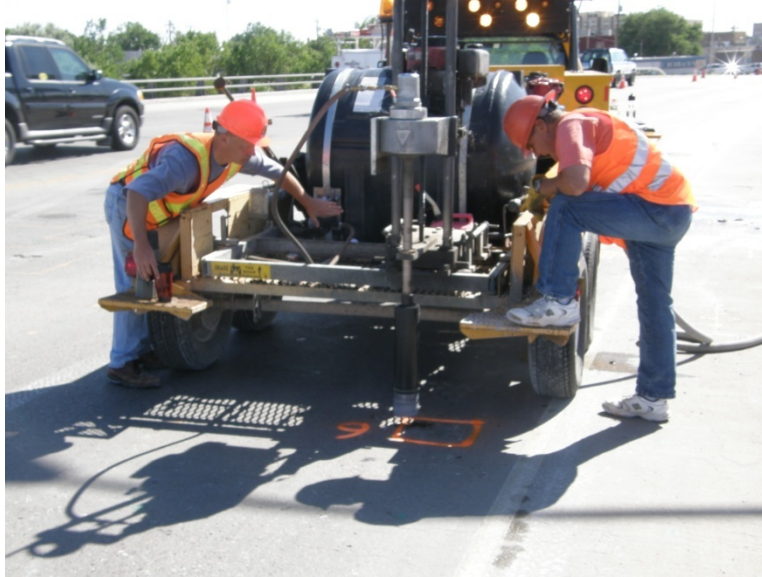
Figure 28: Coring rig on Casper Bridge.
