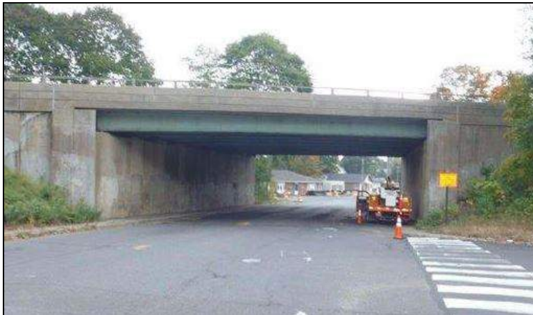
Bridge 00579 (1956) carries Route 8 over Division Street in Ansonia.
