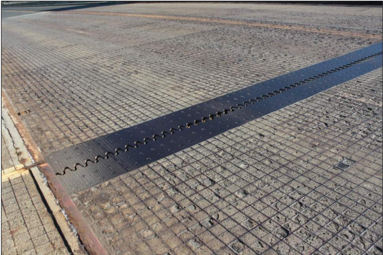
Detail of roadway joint between bascule leaves, camera facing southeast.
