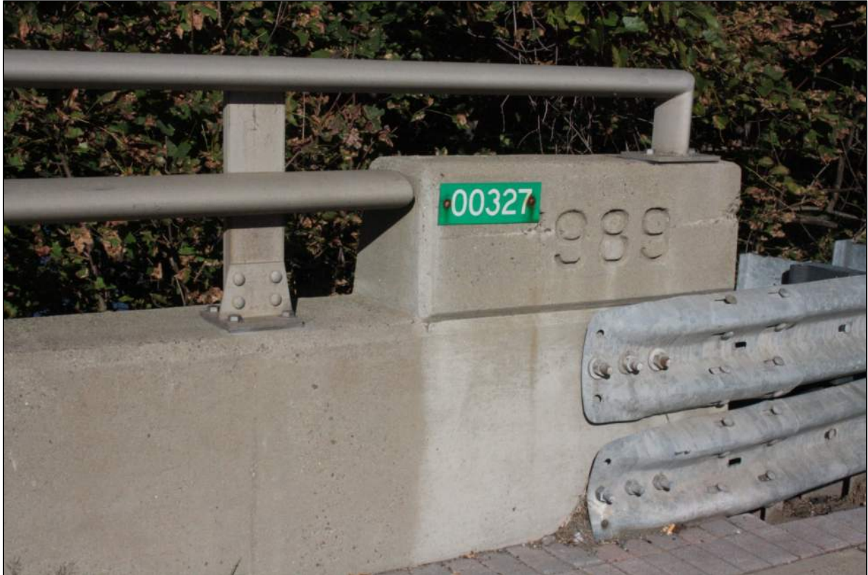
Detail of end of north parapet, camera facing northeast.
