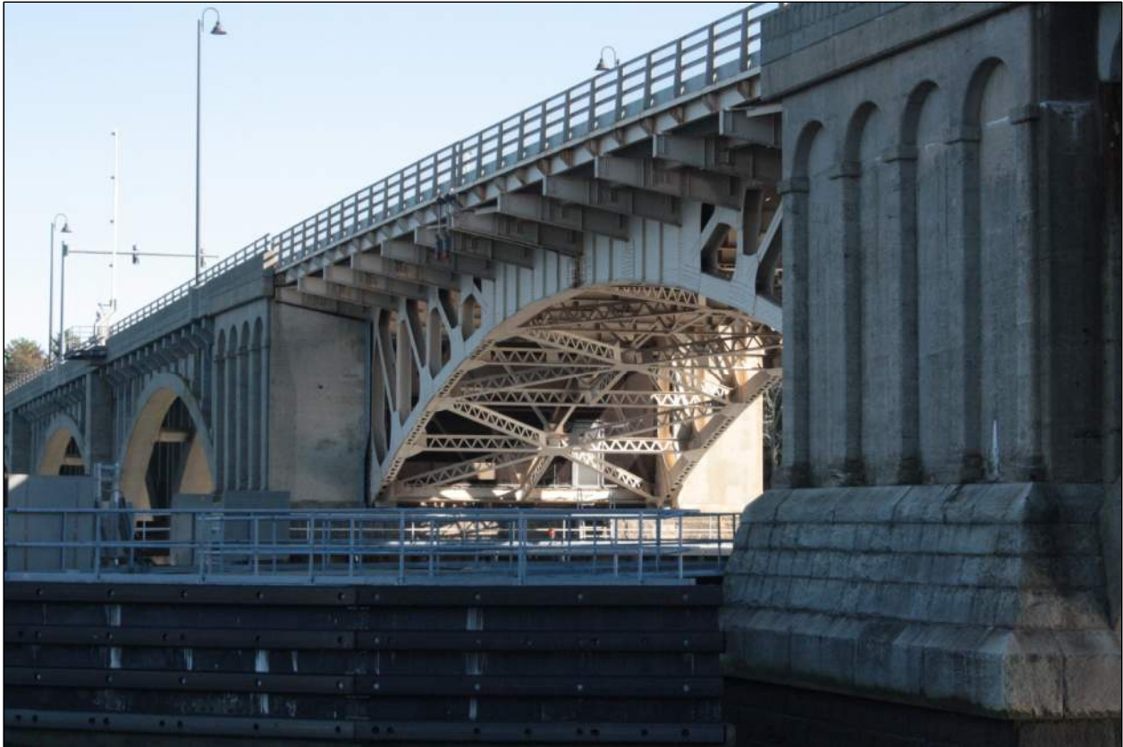
Closer view of double-leaf bascule, north elevation, camera facing southeast.
