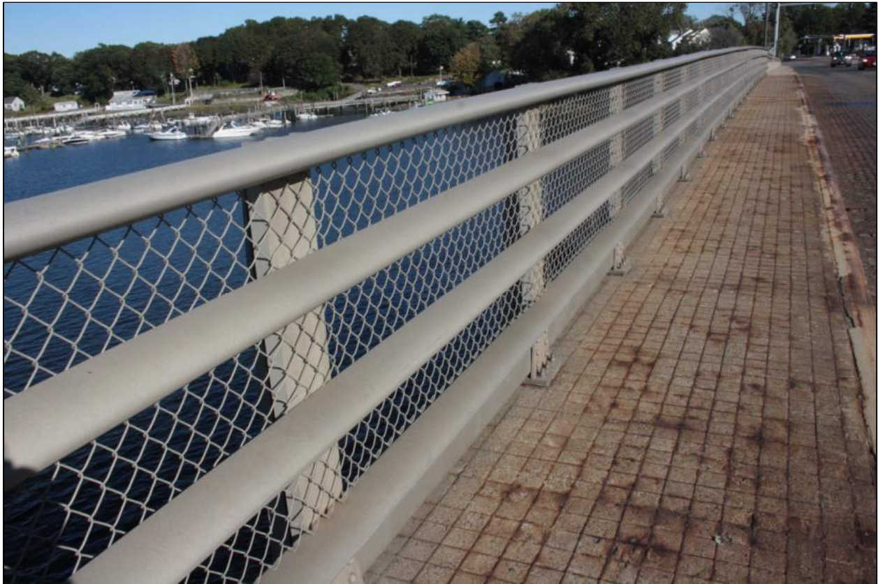
Detail of railing and sidewalk, camera facing east.
