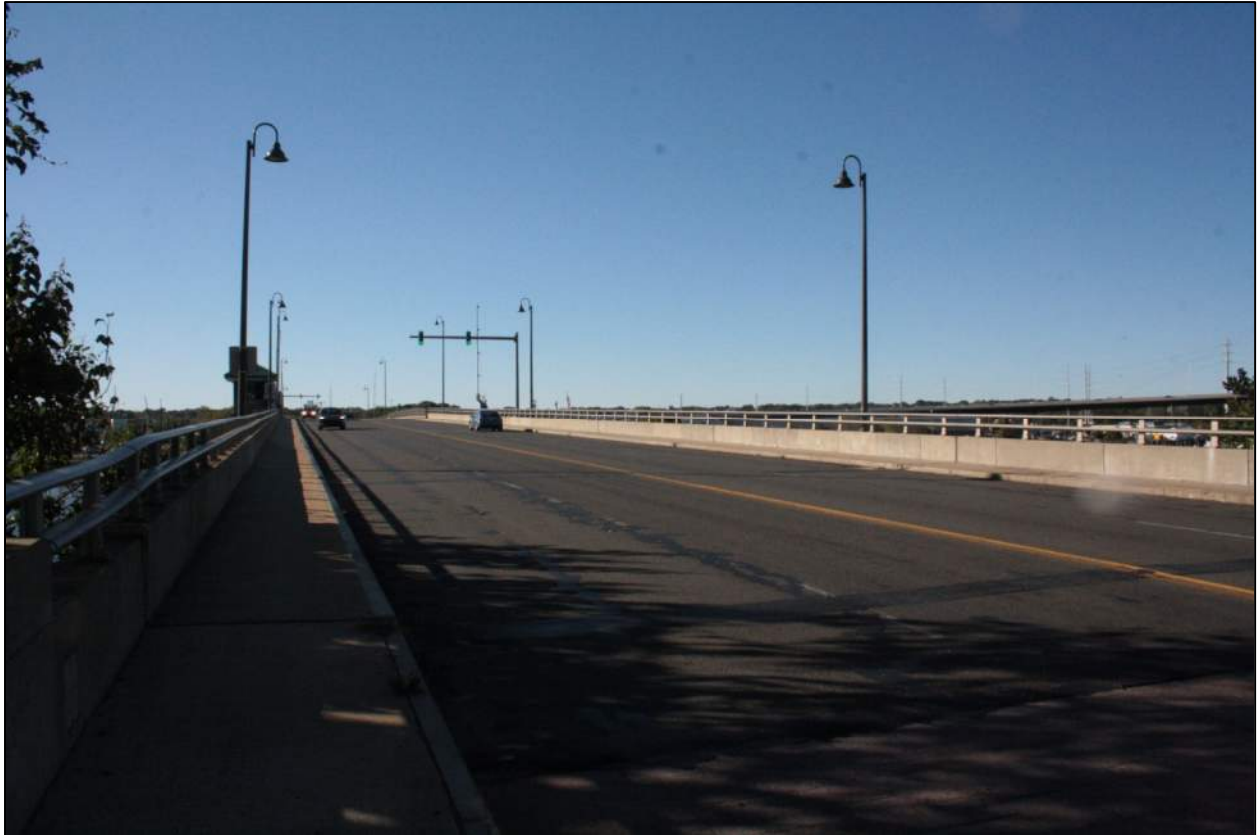
Roadway level from east end, camera facing northwest.
