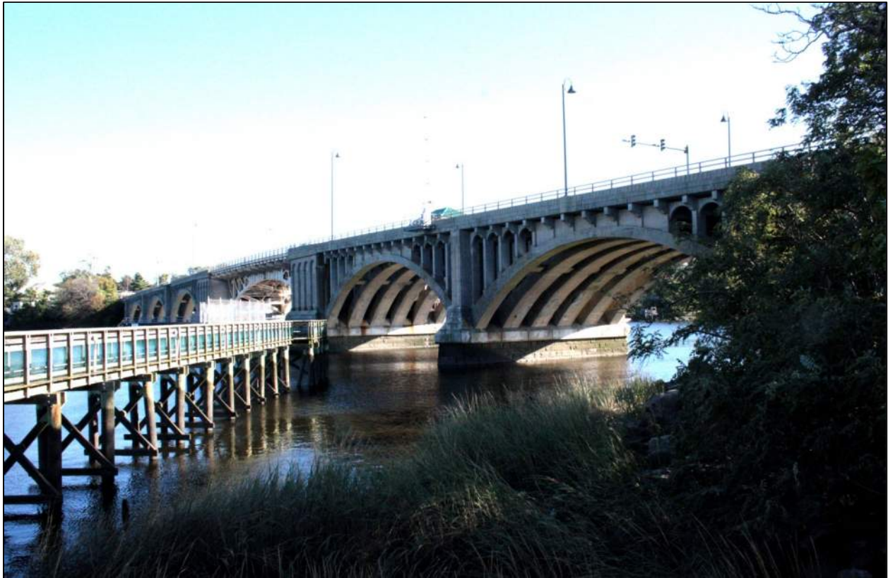
North elevation, camera facing southeast.
