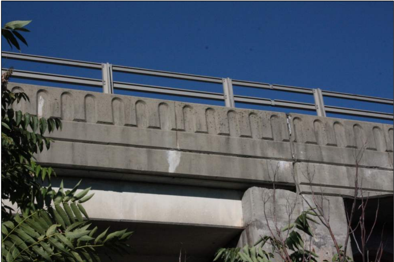
Detail of outside of south parapet, camera facing north.
