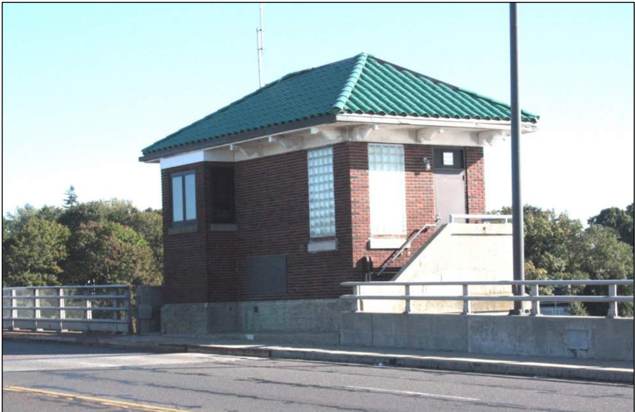
Detail of west operator house, roadway side, camera facing southeast.
