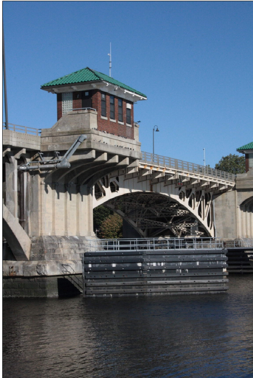
Detail of west operator house, river side, camera facing northeast.
