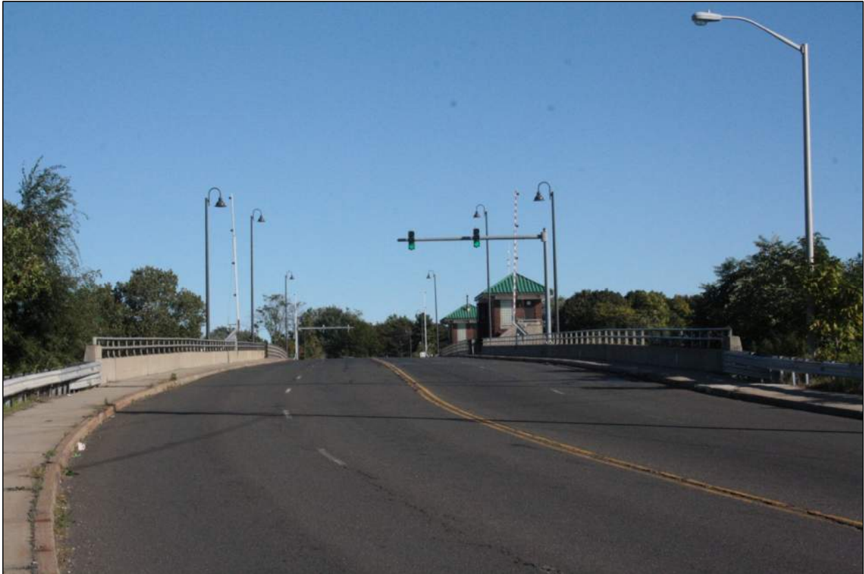
Roadway level from west end, camera facing east.
