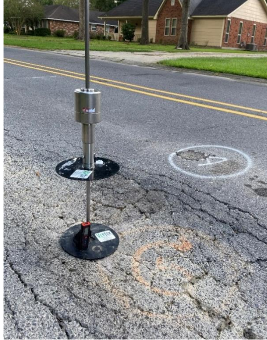
Figure 28. Photo of Zone 10 DCP and core location
