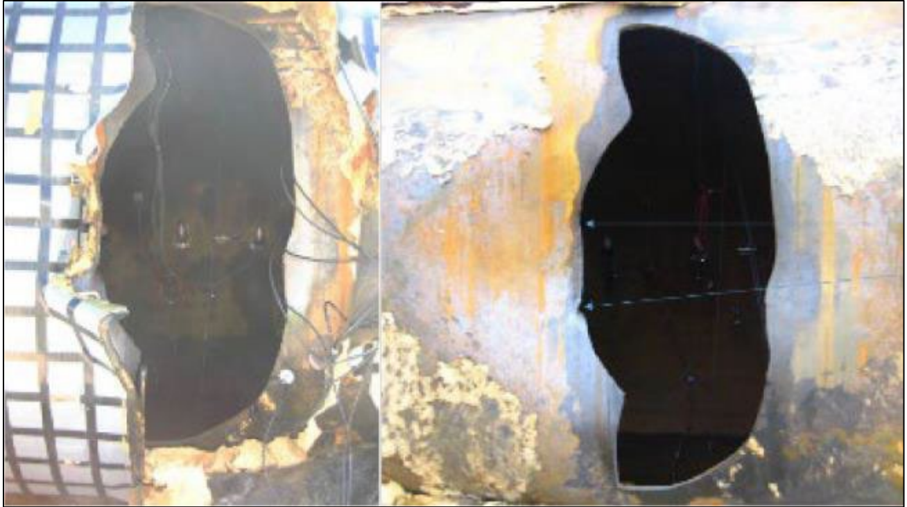
Figure 56. Test 6 – Impact Zone Post-testing (left) With and (right) Without Jacket
