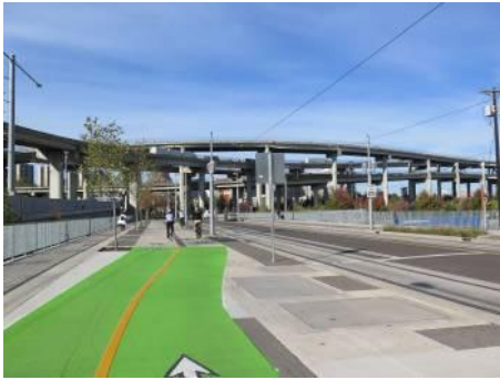
2-way green lane sidepath
