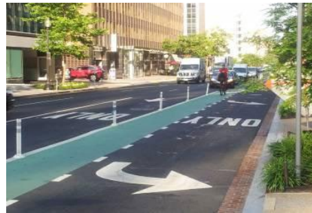
Green bike lane between through and left turn lane on urban street
