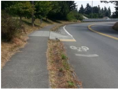
Merging ramp onto roadway
