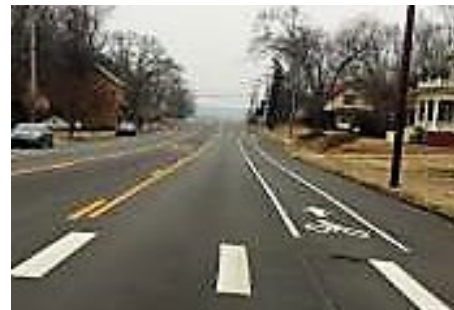
Bike lane on road with 2 motor vehicle lanes, center left turn lane
