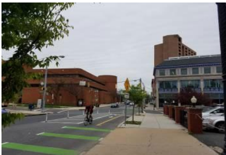
2-way separated bike Lane on urban street
