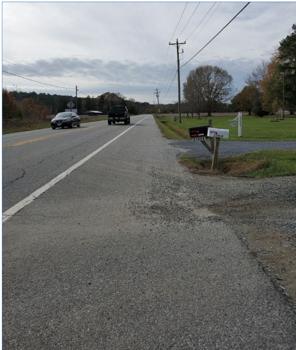
Figure 65. Driveway Gravel Impacts Surface Quality for Cyclists
