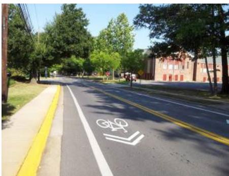
Shared lane marking
