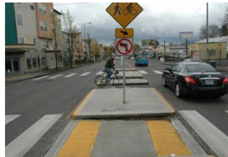
Crossing with median refuge island
