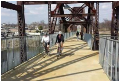
Multi-use trail bridge
