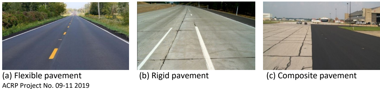
Figure 1. Three typical types of pavements
