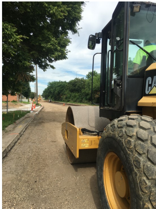
Figure 77. Intelligent compaction on top of subgrade and base layers in the field
