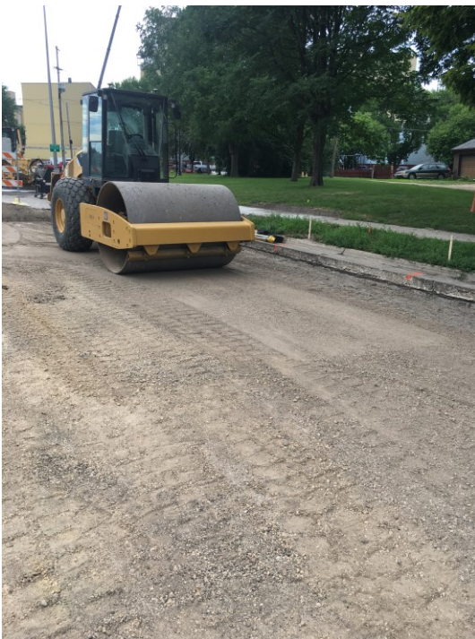
Figure 77. Intelligent compaction on top of subgrade and base layers in the field
