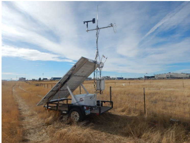
Figure 10: Installed system near exit 4 on I-25 (MP 4.5)
