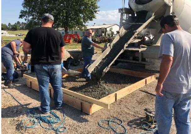
Figure 3 - Casting the 6' x 6' slab with 47BD concrete Salt Valley's maintenance yard
