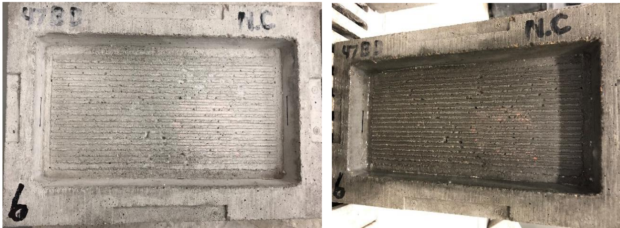
Figure 15 - B6 before testing (left) and after testing showed little signs of scaling after 85 F-T cycles.
