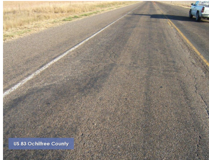
(a) Condition before CIR construction
