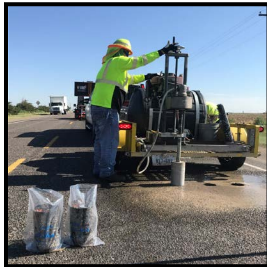
Figure 19. FWD and Coring of existing CIR Section.
