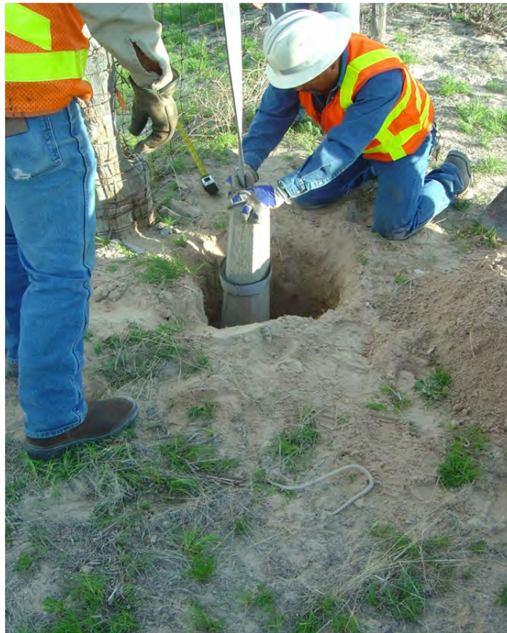
Figure 7.13: Placement of new ROW marker in the existing location of the deteriorated ROW marker
