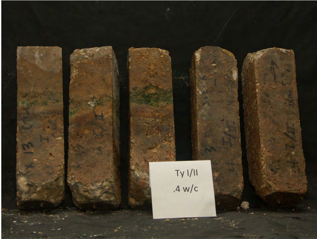
Figure 5.23: Damage to mixtures with Type I/II binders at a 0.4 w/cm in sodium sulfate exposure
