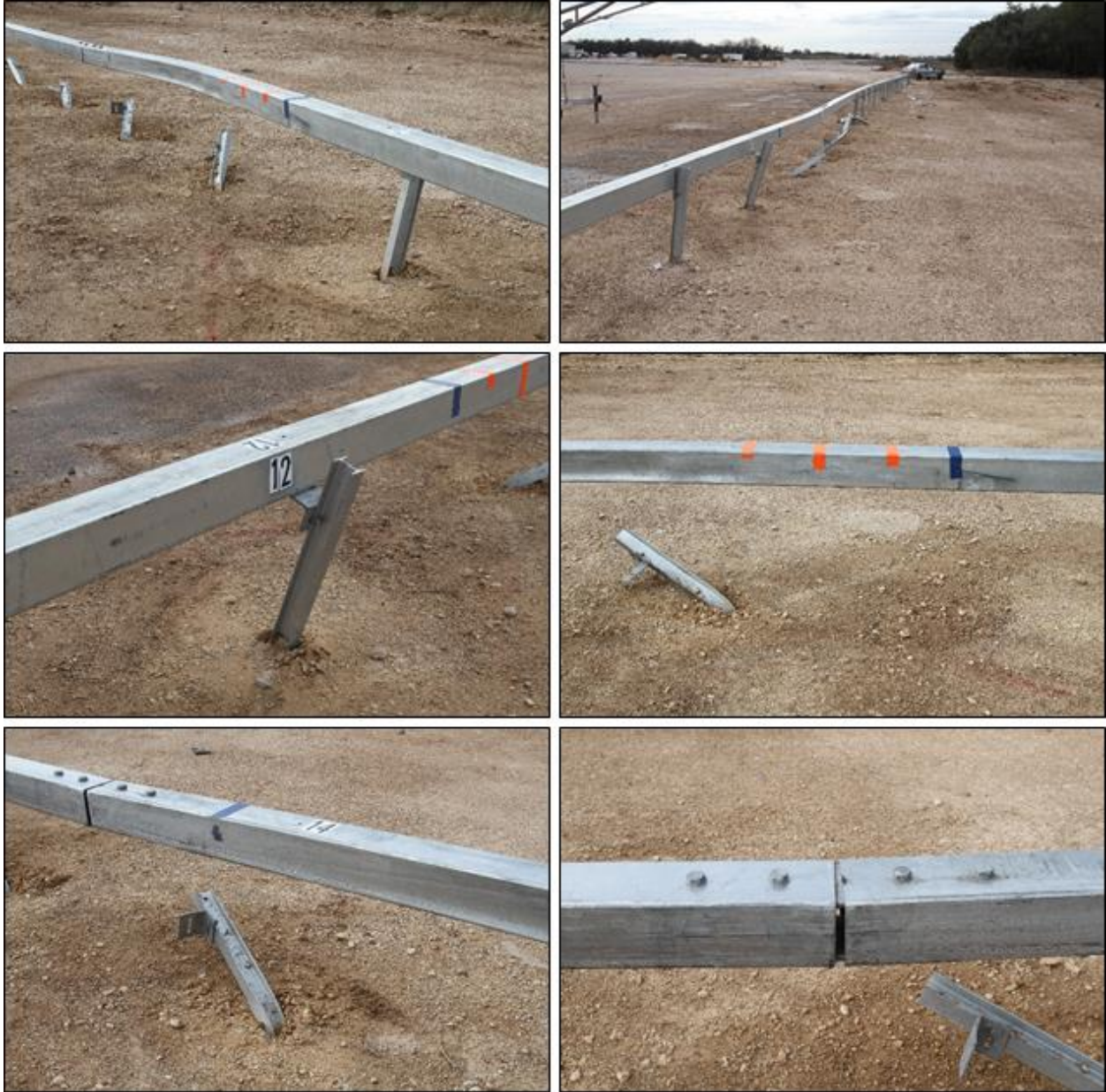
Figure 5.4. Damage at Impact Area after Test No. 610031-01-1.
