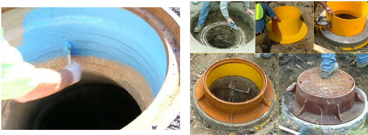
Figure 23. (a) application of Flex Seal Utility Sealant; (b) installation of I&I Barrier.
