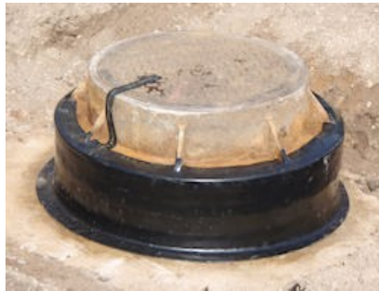
Figure 12. Infi-Shield Uni Band installed on manhole casting.
