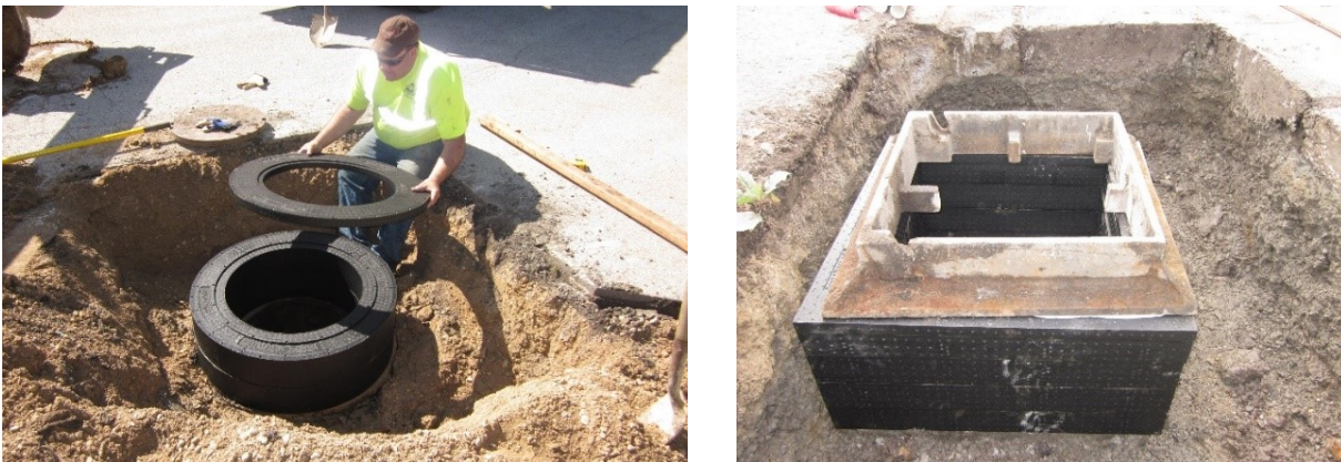
Figure 11. Installation of (a) circular and (b) rectangular (with frame) EPP rings
