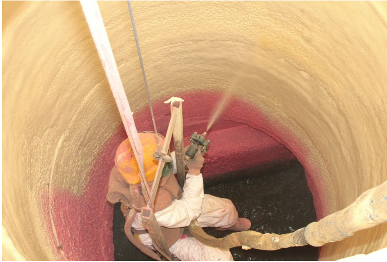
Figure 10. Application of SpectraShield in a manhole.
