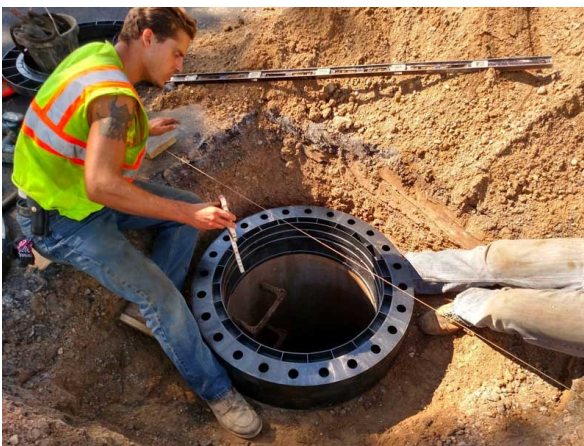
Figure 18. HDPE ring being installed.
