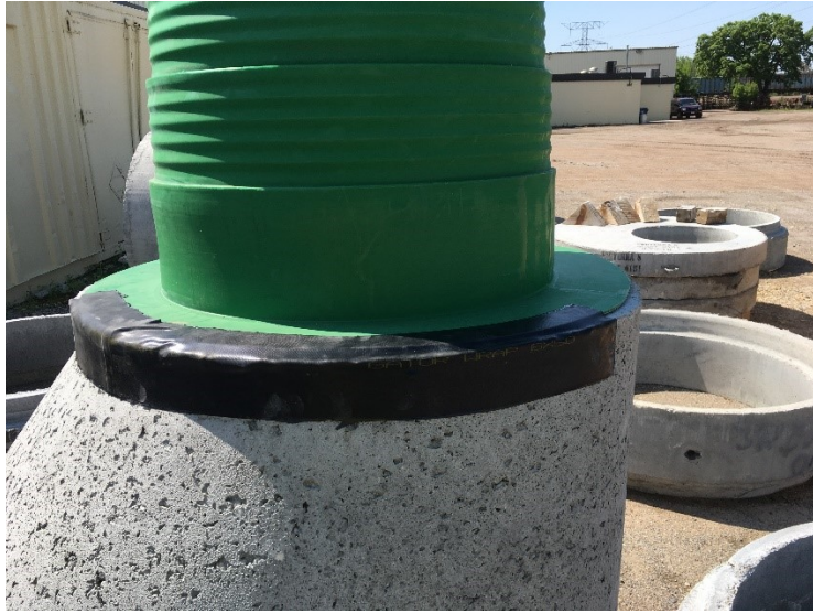
Figure 15. Alignment Barrier on cone with Gator Wrap placed around part of the flange.
