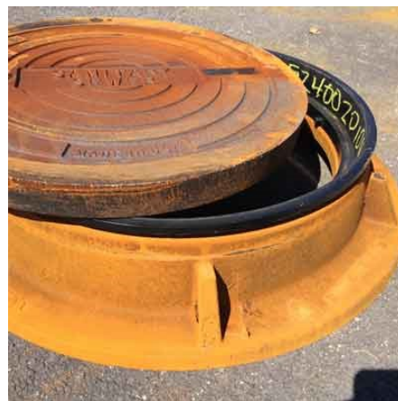
Figure 19. Steel riser ring installed in manhole frame.
