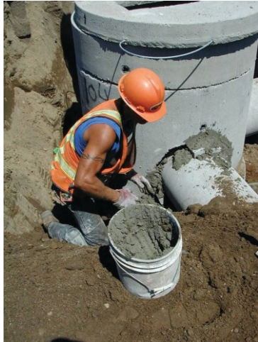
Figure 7. Application of underground utility mortar.
