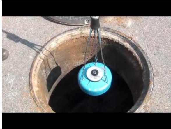
Figure 22. Televising device entering manhole.
