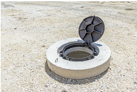
Figure 16. Compacted backfill surrounding manhole.
