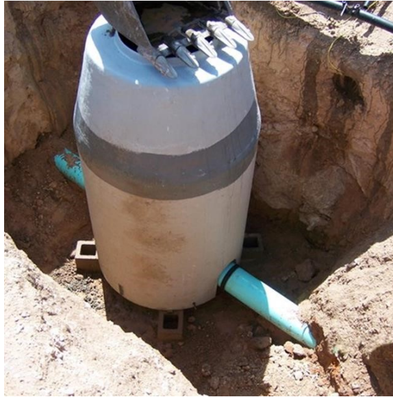
Figure 25. New manhole structure before backfilling.
