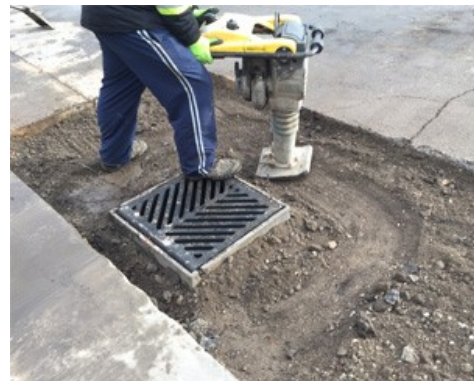
Figure 17. Vibratory plate compactor being used to compact backfill around catch basin.
