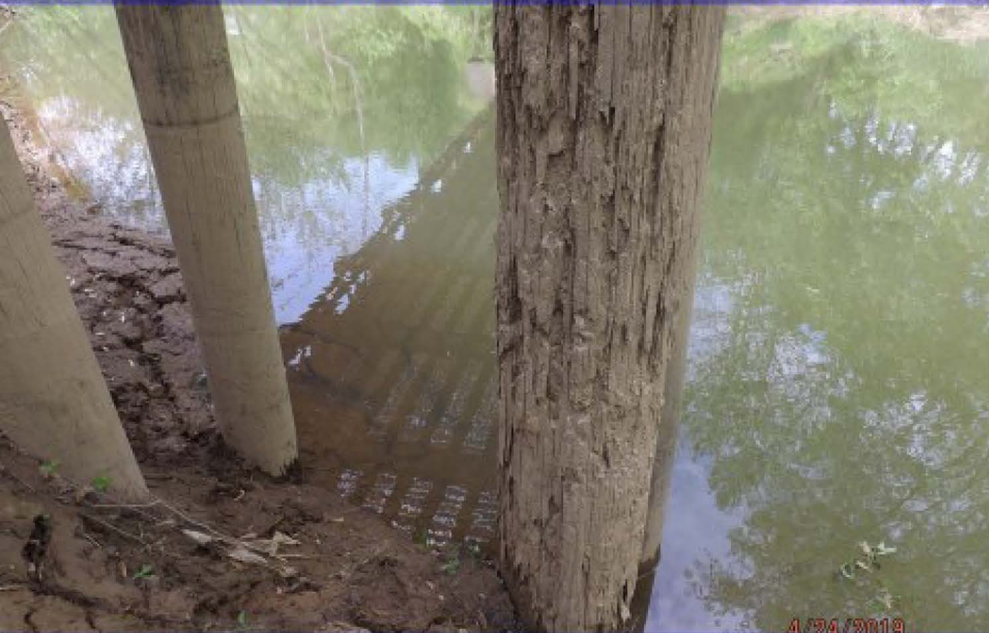
Pier 3: Damage to Timber Pile
