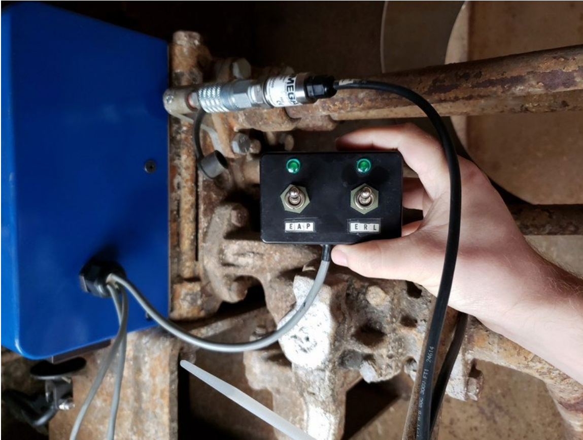
Figure 19 – BCP Fault Switchbox Connected to Emulator on Test Car #1
