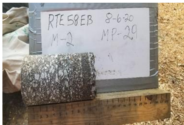
Figure 3. Intact Core on Rte. 58 EB, Richmond District
