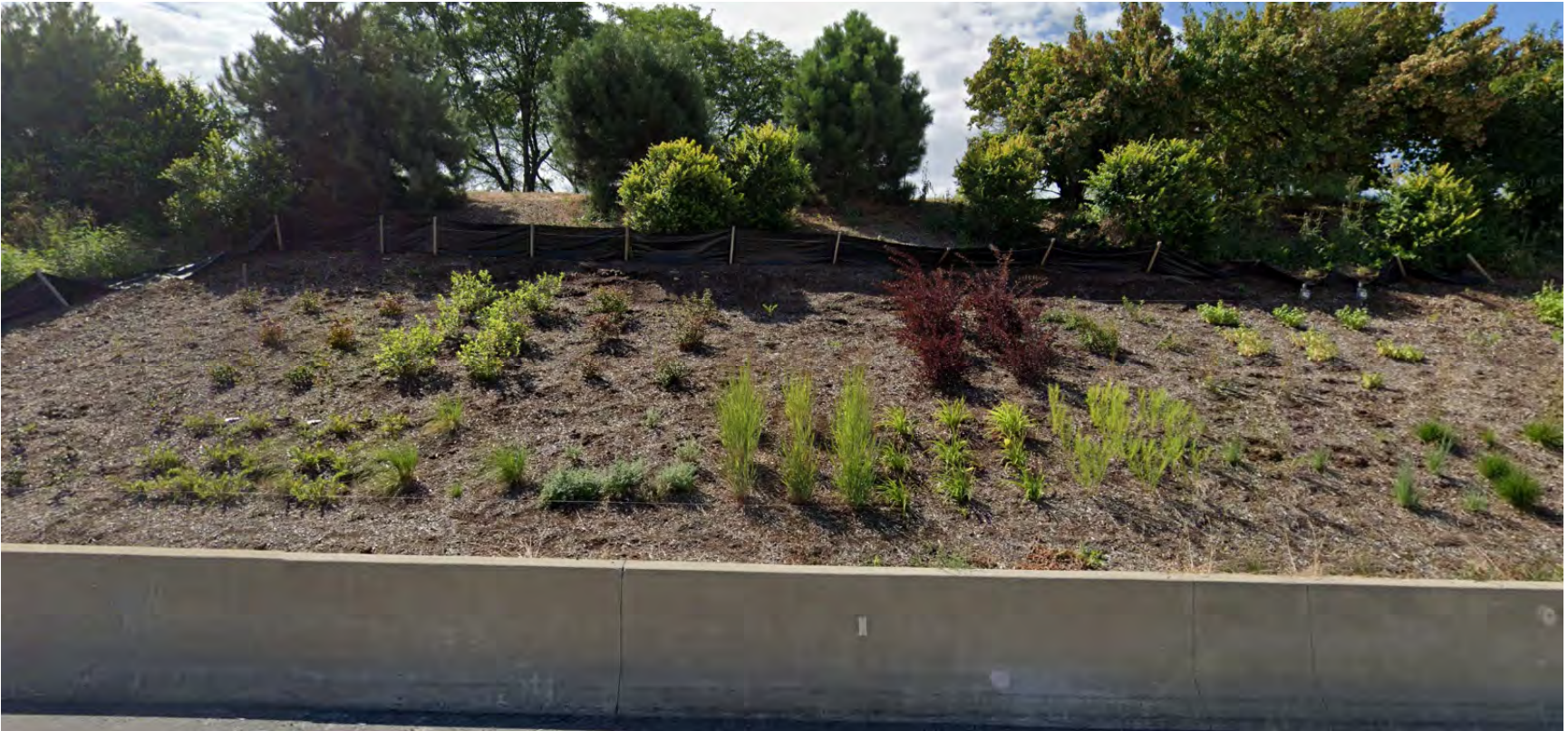
Figure 8. A single treatment plot after plant installation.
