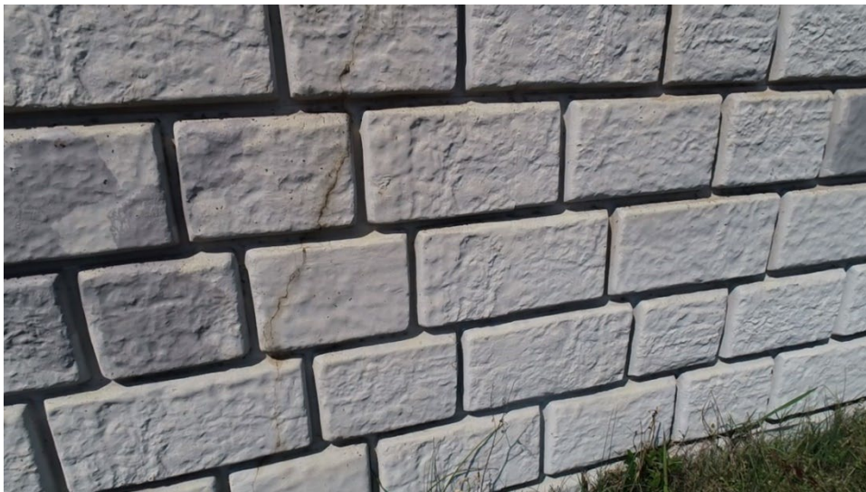
Figure A. 6 Moderate cracks observed on the face of the wall blocks
