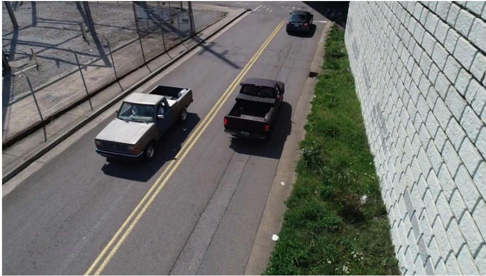
Figure A. 5 Fairly good vegetation at the foot, no soil erosion and deflection/displacement observed
