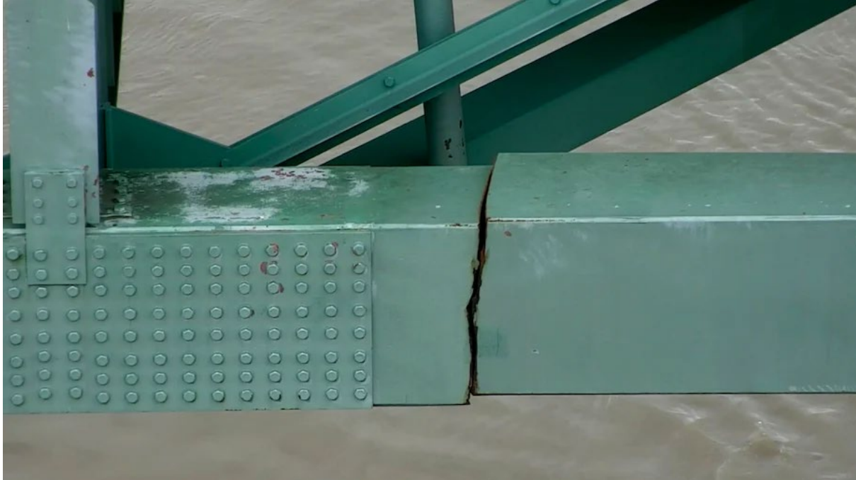
Figure 1-1. A detected crack in a critical steel support beam of the I-40 Bridge.
