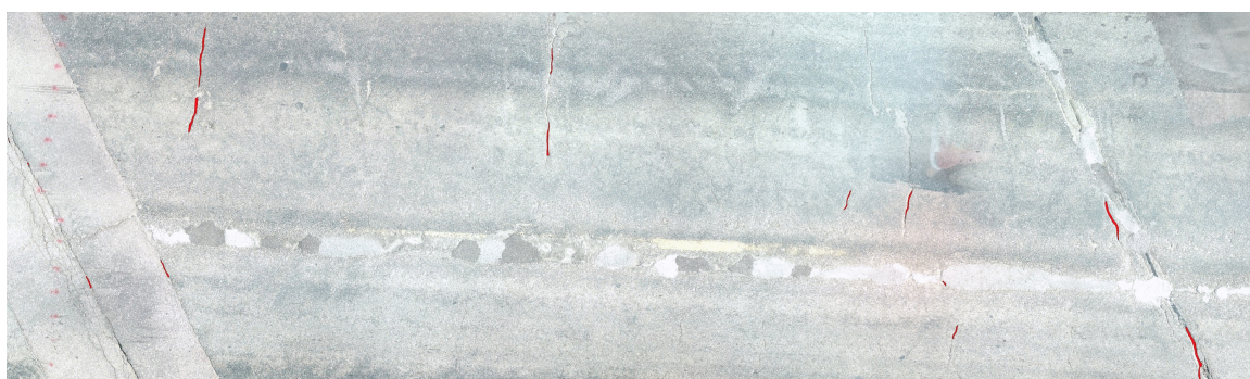
(b) Closeup view of the left top corner with cracks detected on Bridge S075 17596 (asphalt overlaid concrete deck)
