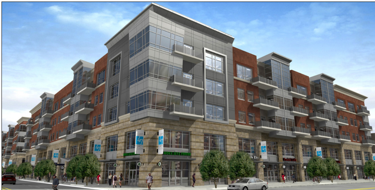
Figure 15. Completed Mixed-Use Structure
