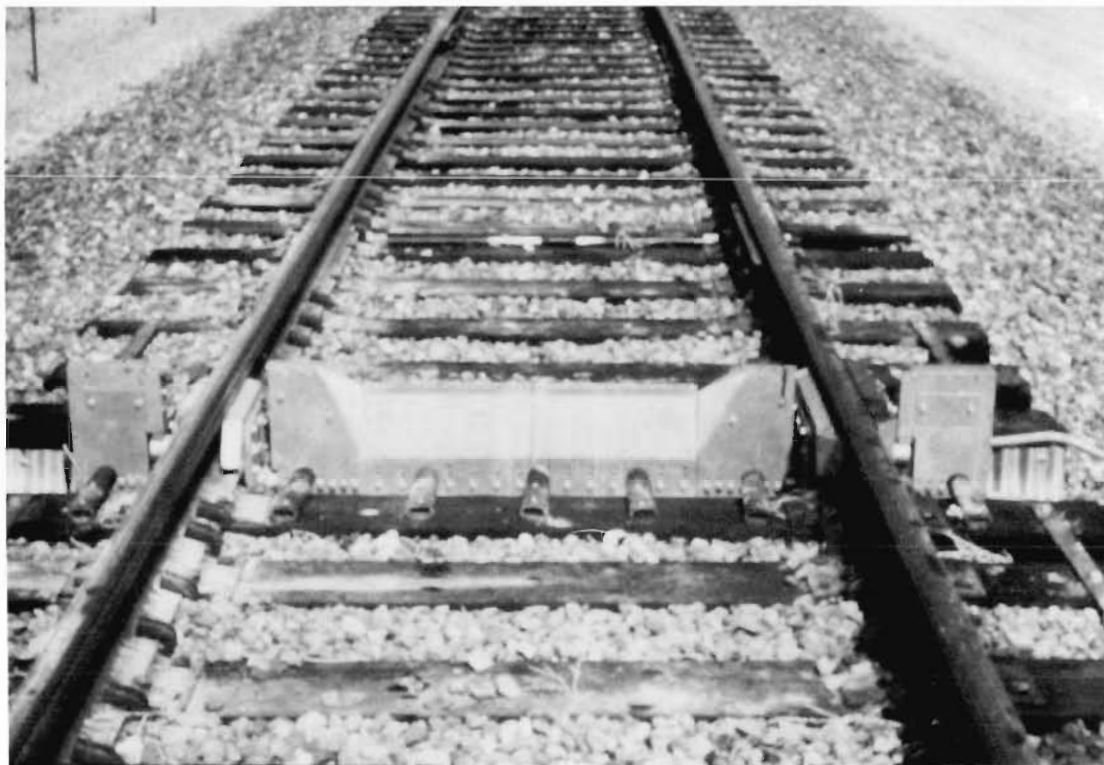
DRAGGING EQUIPMENT DETECTOR
