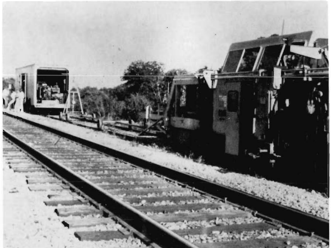
THE WES'S TRAILER-HOUSED VIBRATOR ON-SITE ON THE ROCK ISLAND RAILROAD IN ARKANSAS
