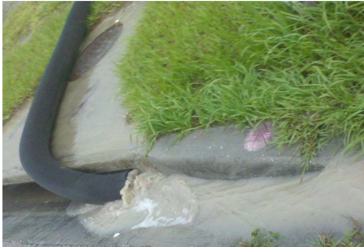
Figure 4: Improper curb inlet protection practice
