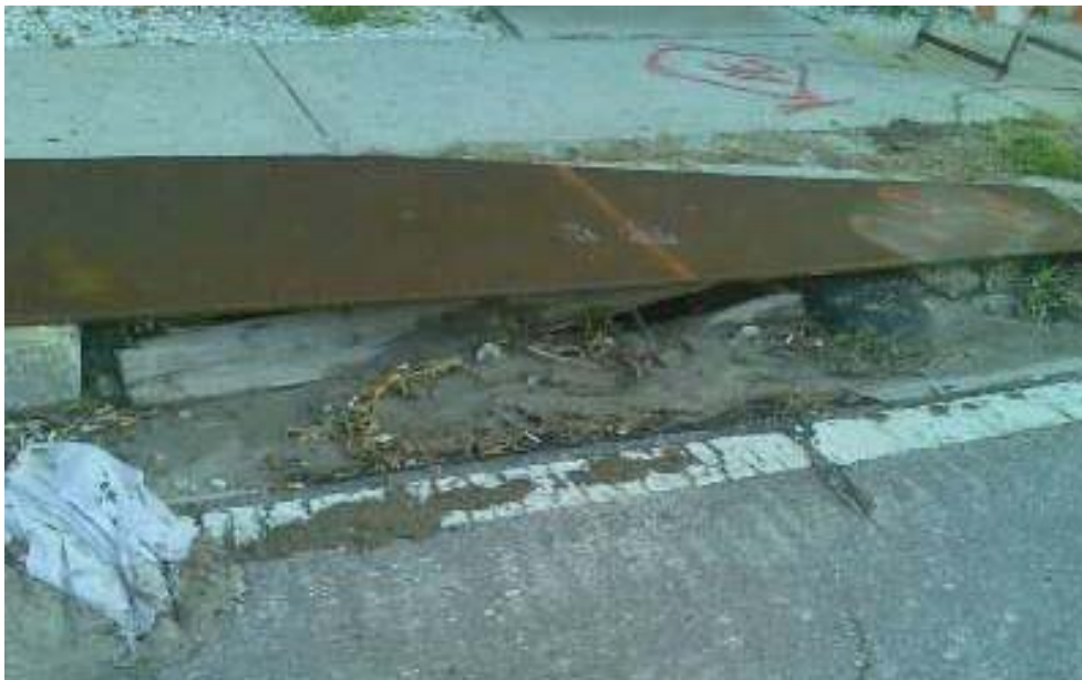
Figure 1: Lack of inlet protection
