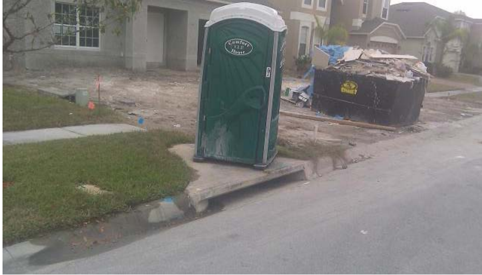
Figure 2: Absence of inlet protection on residential construction
