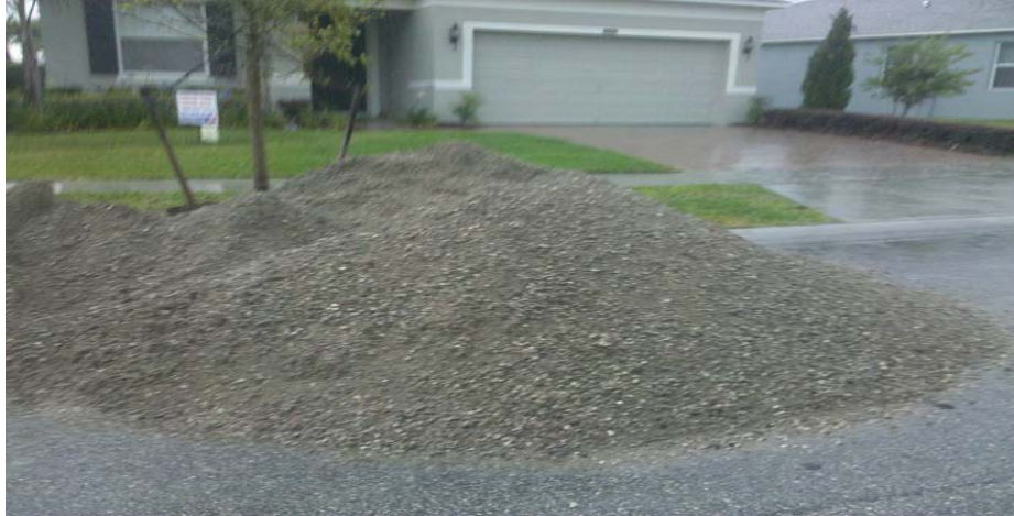
Figure 5: Improper aggregate storage
