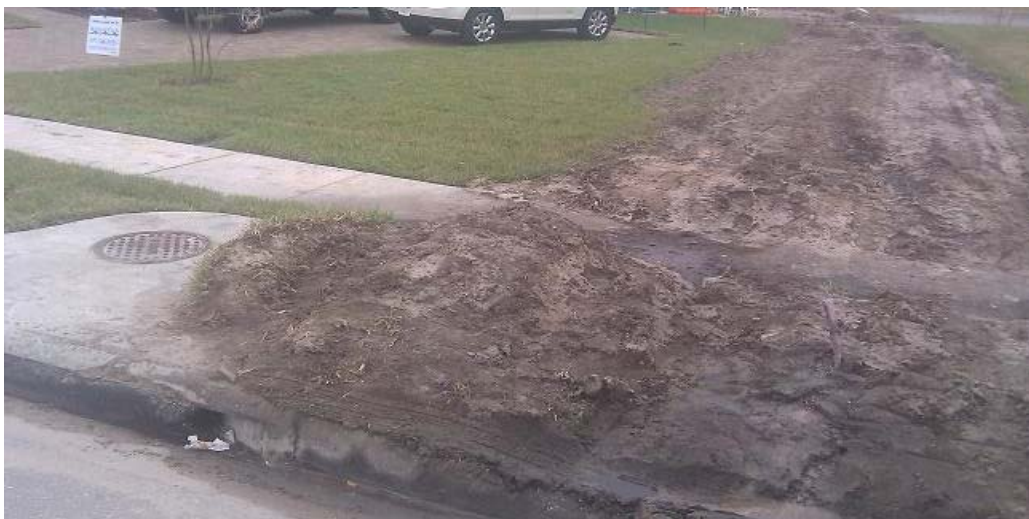
Figure 6: No source control adjacent to inlet
