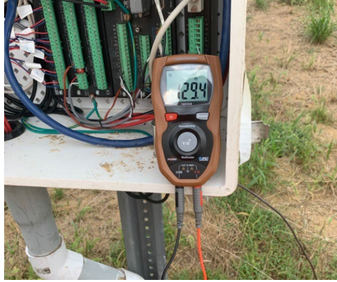
Figure 63. Measurement of the sensors’ resistance prior to testing
