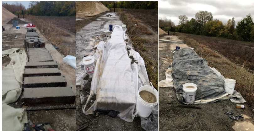
Figure 17. Sample curing and protection on site
