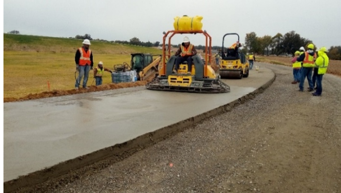
Figure 12. Finishing process
