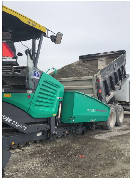
Figure 10. Loading process of the slip-form paving
