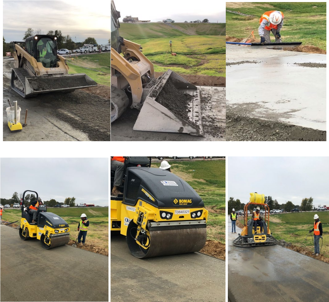
Figure 5. Density adjustments
