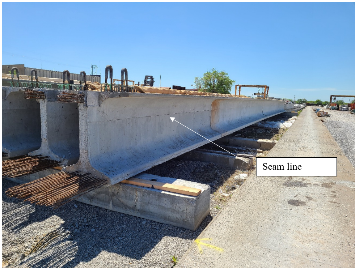
Figure 3-4. Seam line in beam for precast Plant #1
