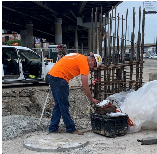
Figure 4-24: CSL testing is performed on the shaft for Ramp F Bent 5.
