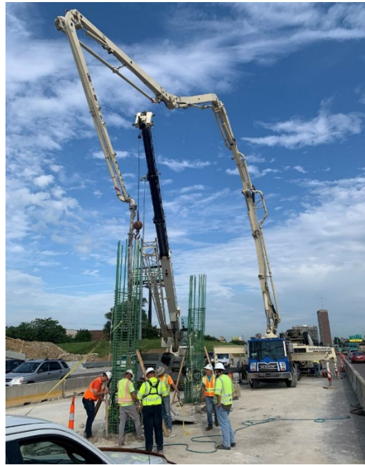
Figure 4-15: Concrete placement for Ewing Ave. Shaft 2.
