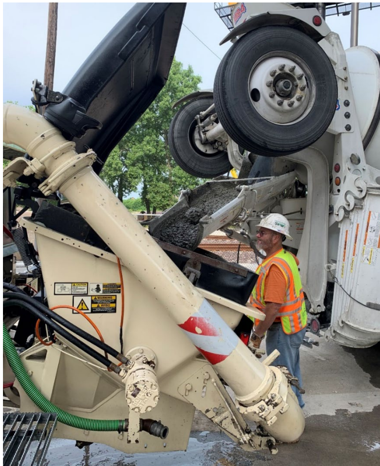
Figure 4-17: Concrete is transferred from concrete truck to pump truck.
