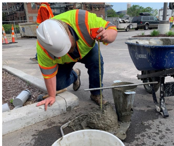
Figure 4-14: Concrete slump test performed for Ramp F Bent 5 drilled shaft.
