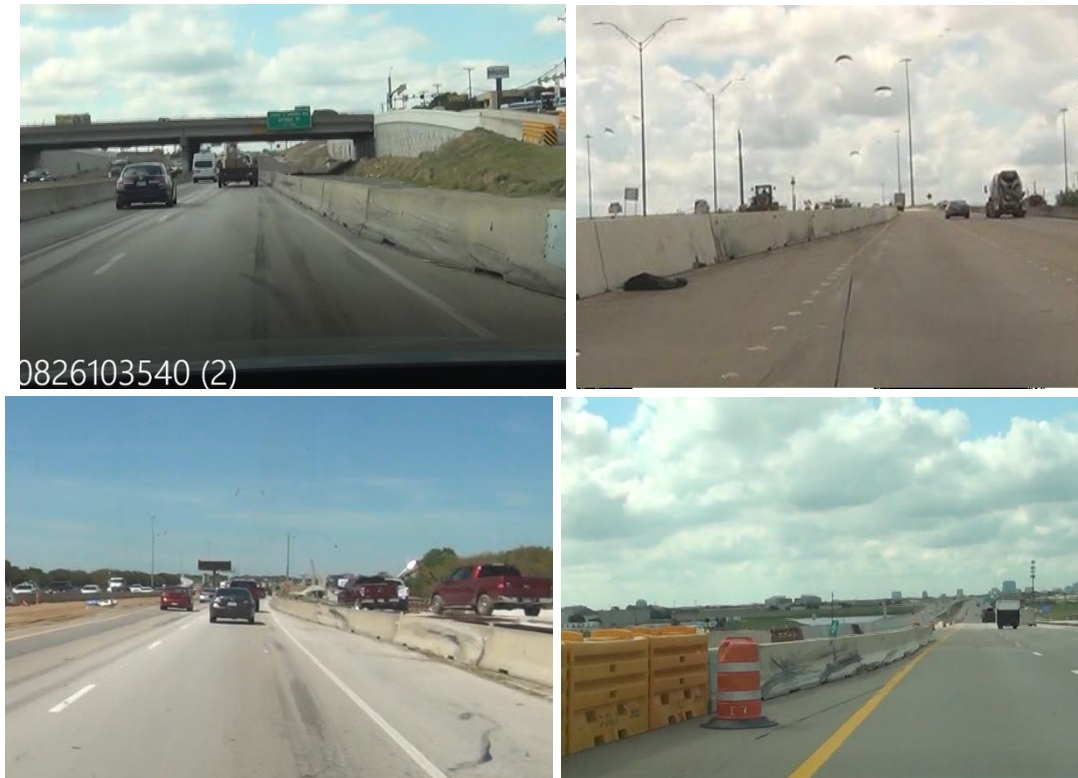
Figure 11. Examples Where Inconsistent Barrier Presence and Offset Distance Are Associated with Increased Tire Scuffs and Impact Scars.
