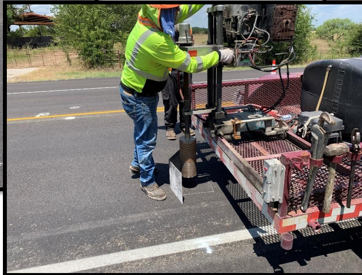
Coring for calibration
