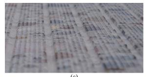
(c) Figure 5. Examples of (a) ground, (b) grooved, and (c) NGCS pavement [32,34].
