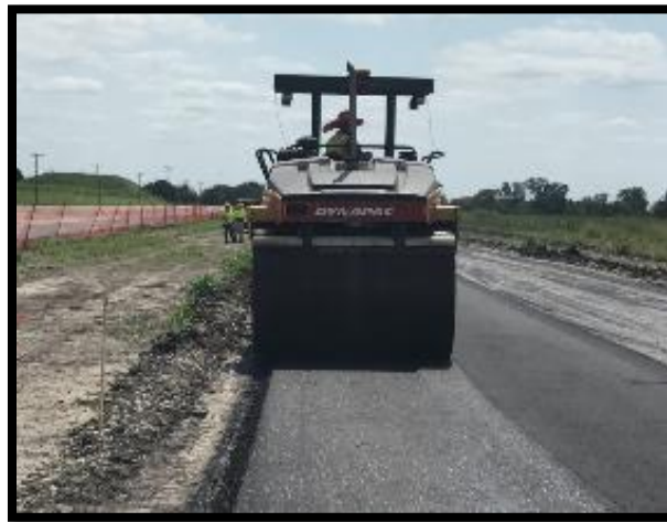
(c) Compaction with CMS system
