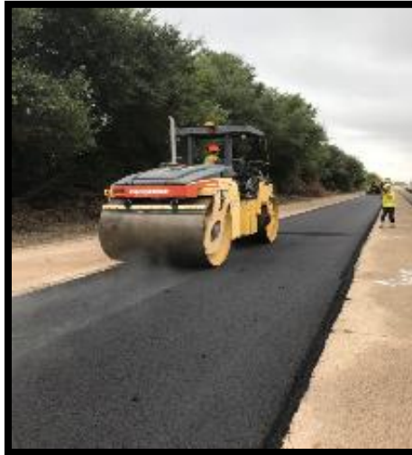
(c) Compaction with CMS system
