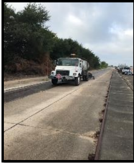
(a) Tack coat application
