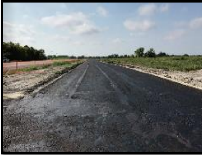
(a) Prime coat applied
