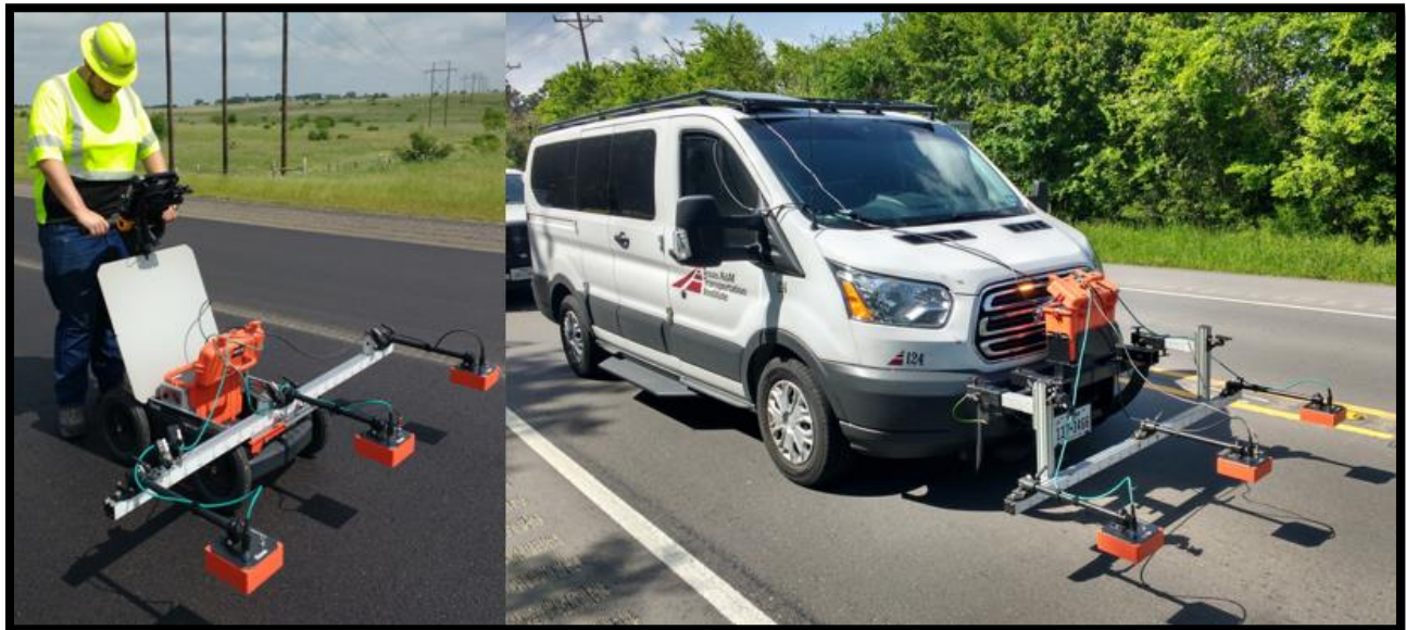
Figure 38. GPR System for Measuring Density of Asphalt Mixture Construction.
