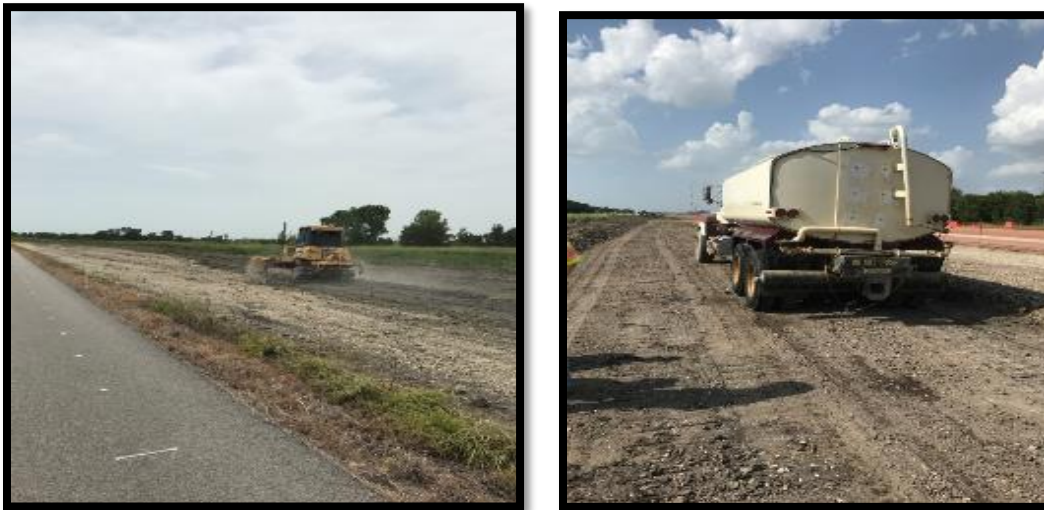
(a) Cleaning and grading
