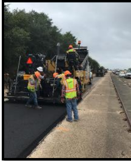
(b) Type-D mix placement
