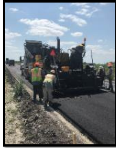
(b) Type-D mix placement
