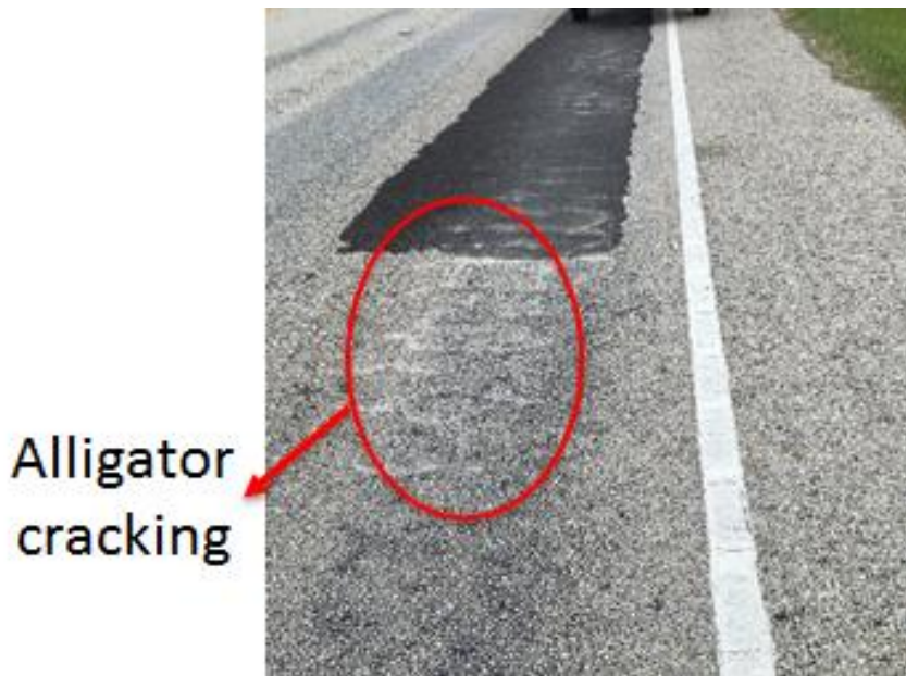
a. Surface Condition of Pavement Section A
