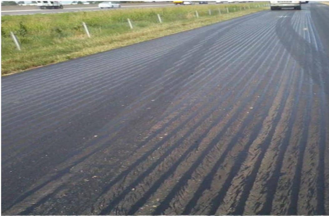
Figure 7-7. Examples of streaks: “Zebra Tack” or “Corn Rows.”
