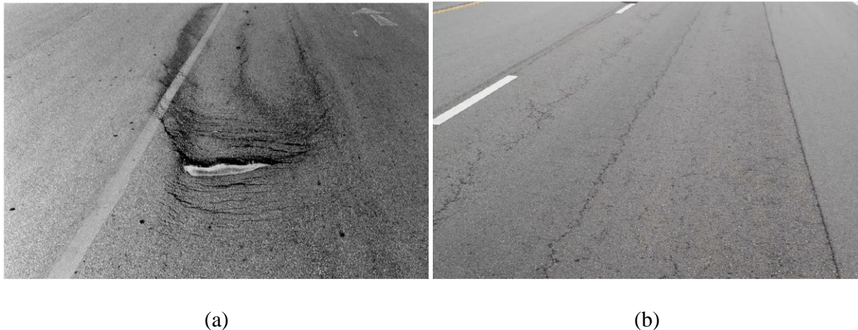
Figure 7-1. Distress due to improper bonding: (a) debonding and (b) fatigue cracking (FHWA 2016).
