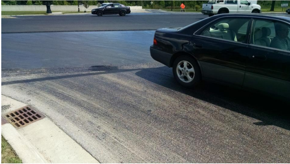
Figure 7-18. Tack coat tracking due to allowed traffic.
