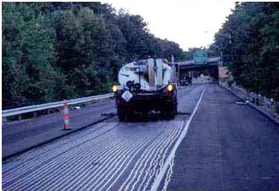
Figure 7-11. Non-uniform tack coat: streaks (Mohammad et al. 2012).
