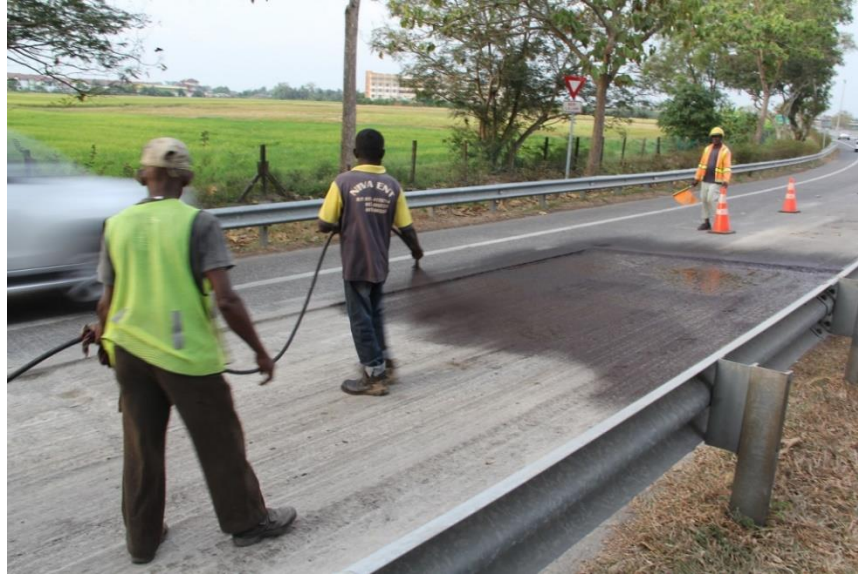
Figure 7-13. Inappropriate use of spray wand to apply tack coat.
