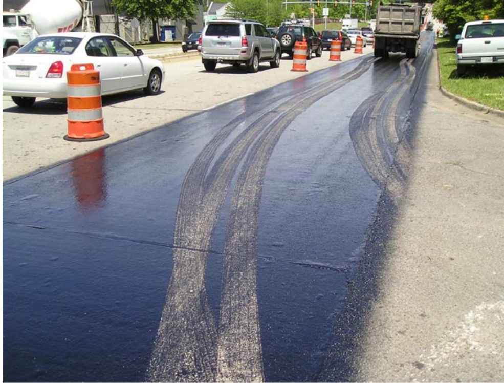
Figure 7-17. Tack coat tracking by haul vehicles in work zone (courtesy: https://roadresource.org/treatment_resources/tack_coat?page=about_process ).
