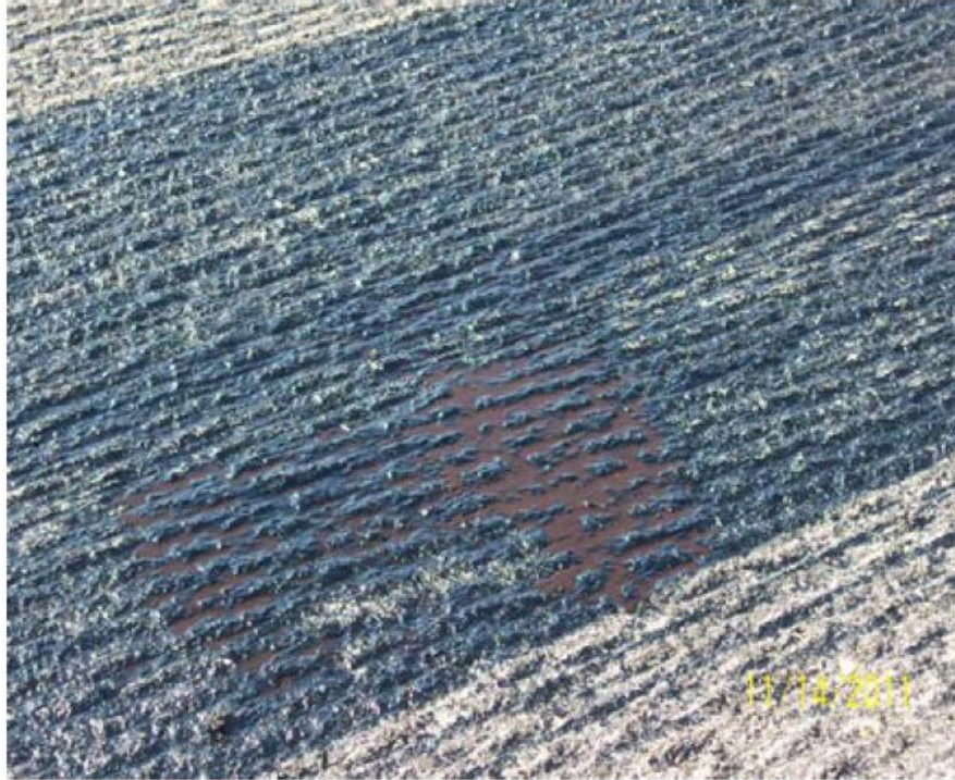
Figure 7-5. Tack coat ‘break’ (FHWA 2016).
