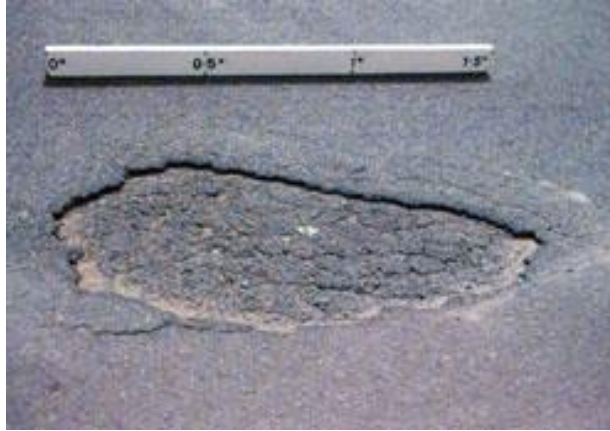
Figure 1-2 Delamination and exposure of underlying layer. (Source: http://www.defence.gov.au/demg/7technical_guidance/aircraft_pavement_manual/part_a/a4.htm )
