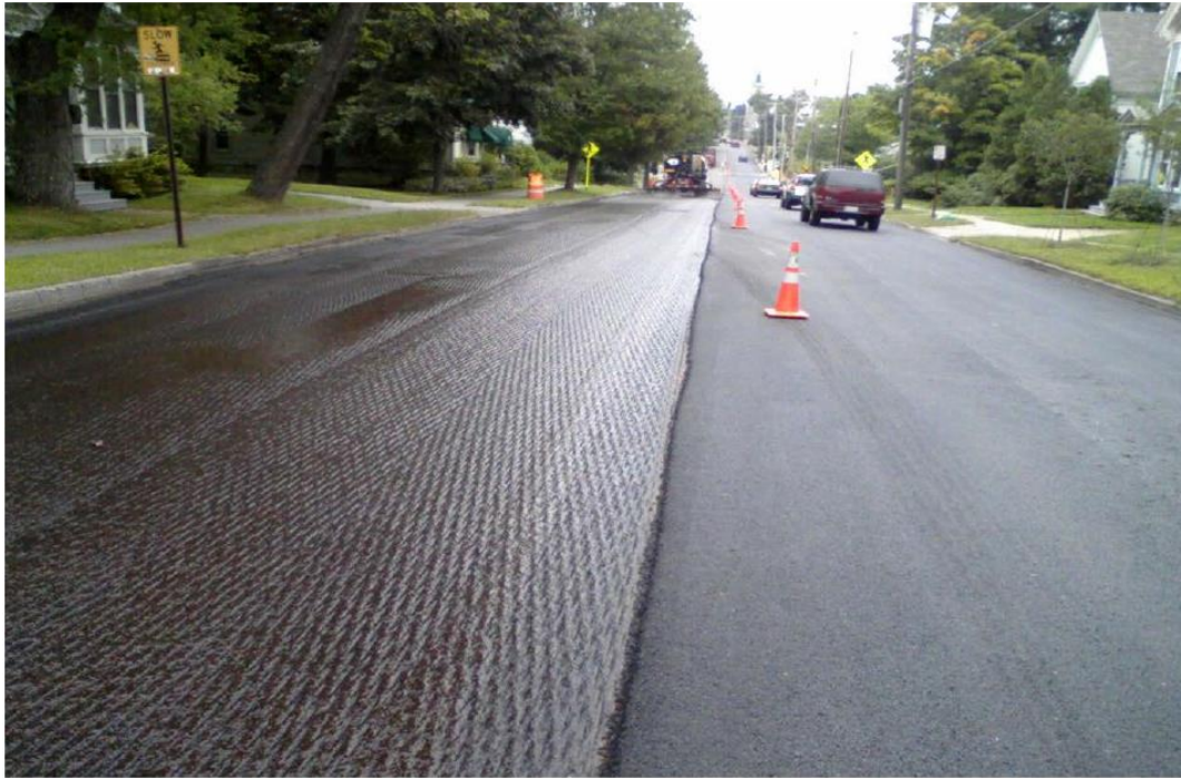
Figure 7-4. Uniform tack application (FHWA 2016).
