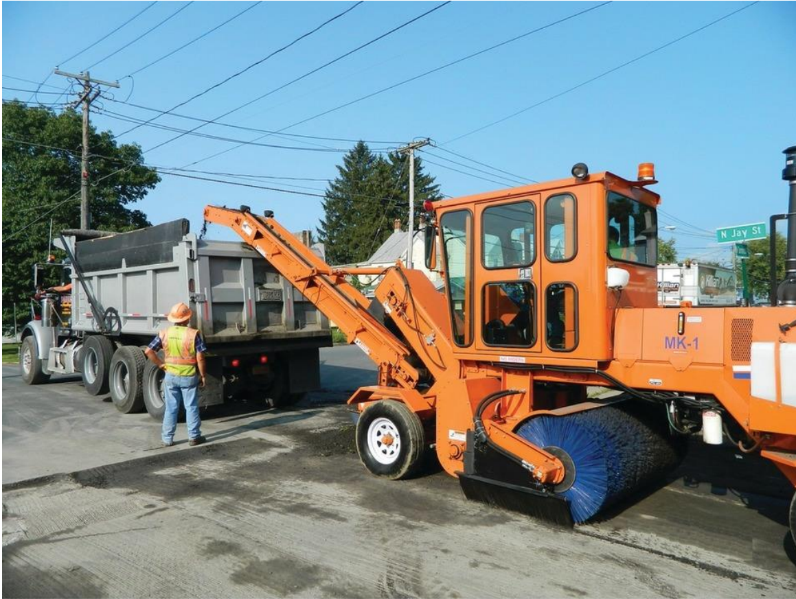
Figure 7-3. Rotary broom eliminating milling debris and loading the truck (courtesy: https://www.forconstructionpros.com/pavement-maintenance/sweepers/article/11237578/how-to-reduce-costly-delays-in-mill-and-fill-asphalt-road-repair ).
