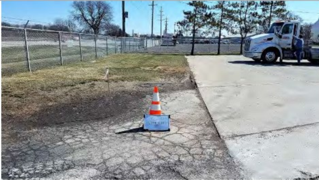
(A) Boring 244-B14, facing east
