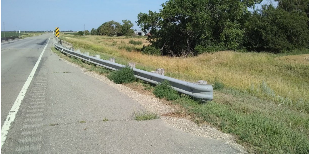
Figure 2.38: Bridge-approach guardrails to Bridge End
