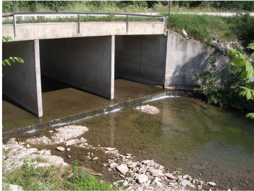
Figure 2.28: Culvert on Rural Road Source: N. Bowers (personal communication, 2019)
