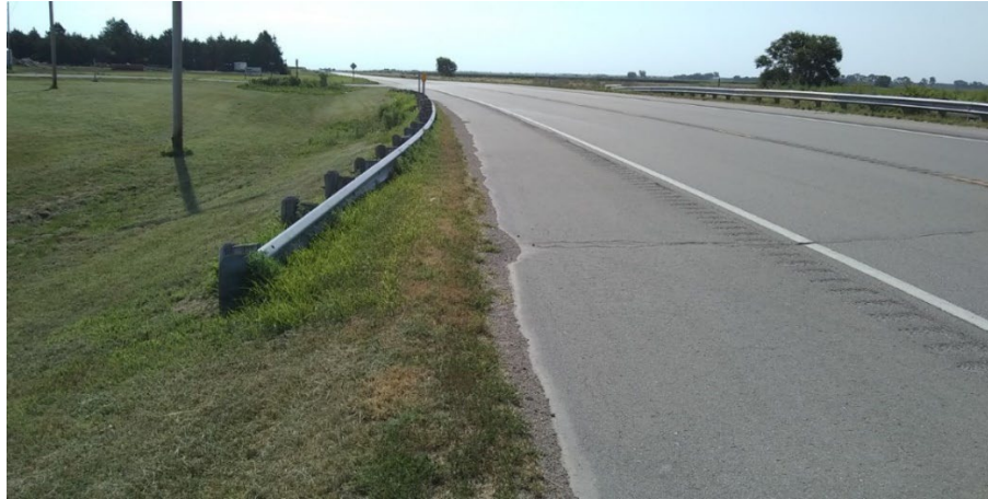
Figure 2.30: Guardrail Shielding a Culvert Source: N. Bowers (personal communication, 2019)
