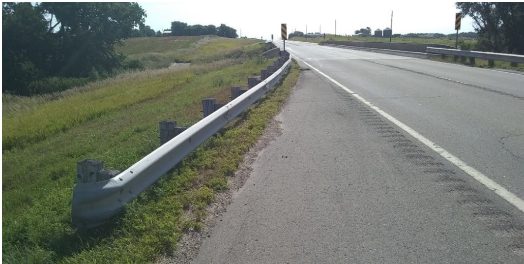
Figure 2.37: Bridge-approach guardrails to Bridge End Source: N. Bowers (personal communication, 2019)
