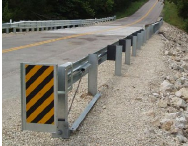
Figure 1.7: Energy-Absorbing Terminal Source: Glennon (2012)
