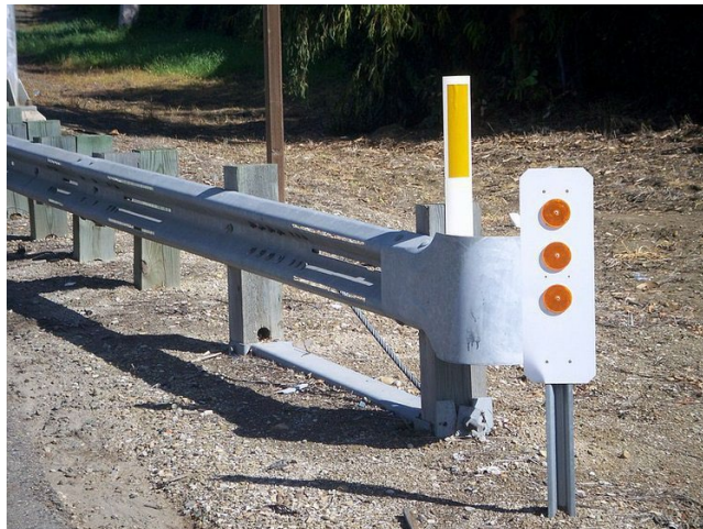
Figure 1.6: Breakaway Cable Terminal
