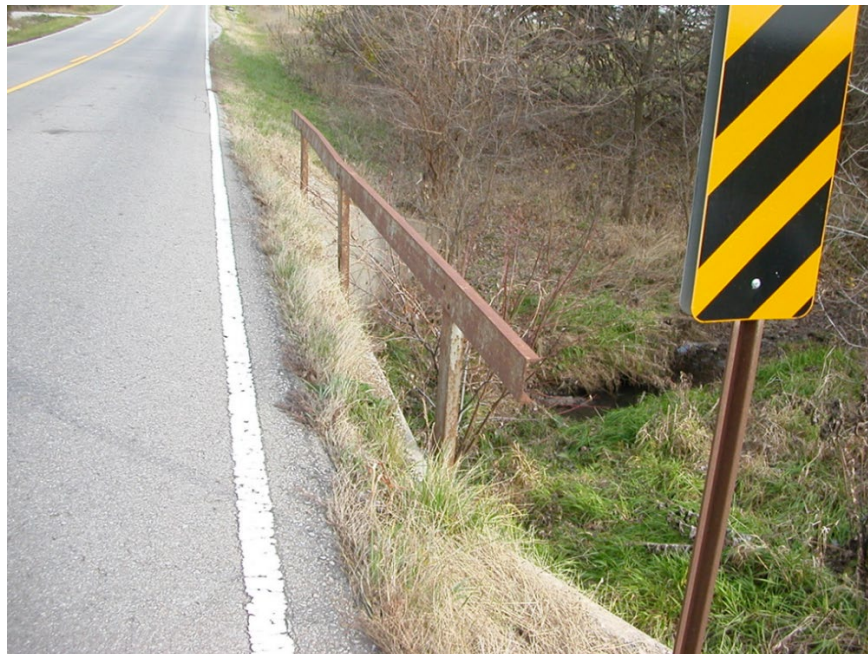
Figure 2.29: Culvert with Zero Offset Source: N. Bowers (personal communication, 2019)
