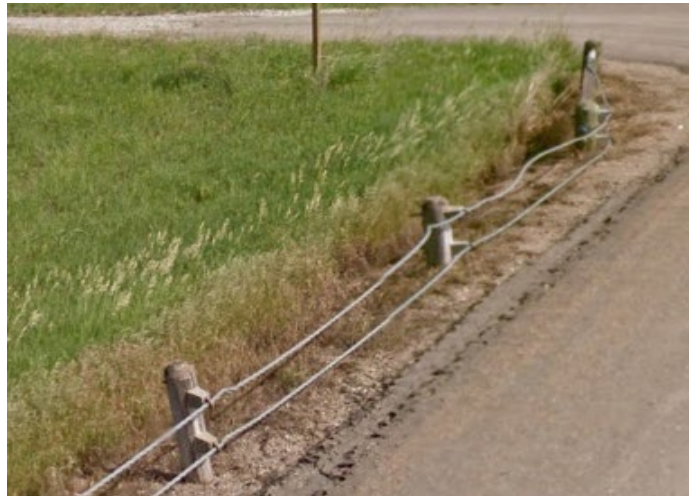
Figure 2.8: Low-Tension Cable Guardrail
