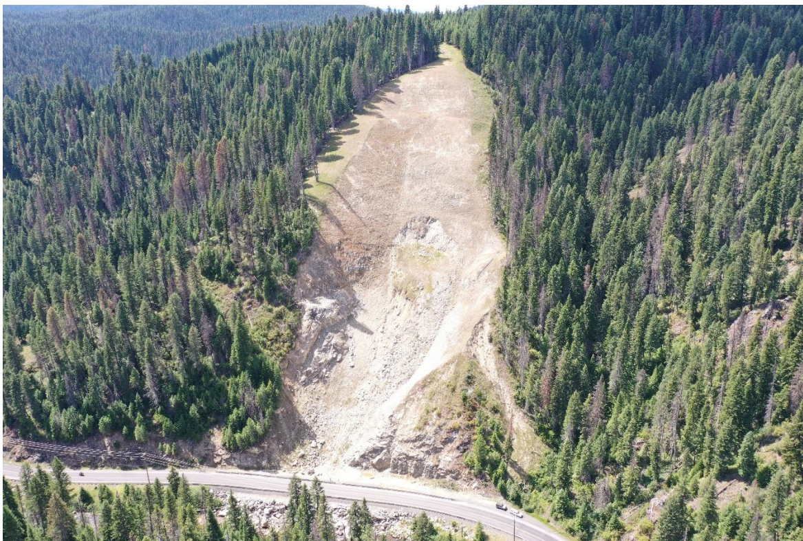
Figure 3.5 Oblique aerial photograph of a landslide along SH-14 west of Elk City (45.828477°N, - 115.584883°E).
