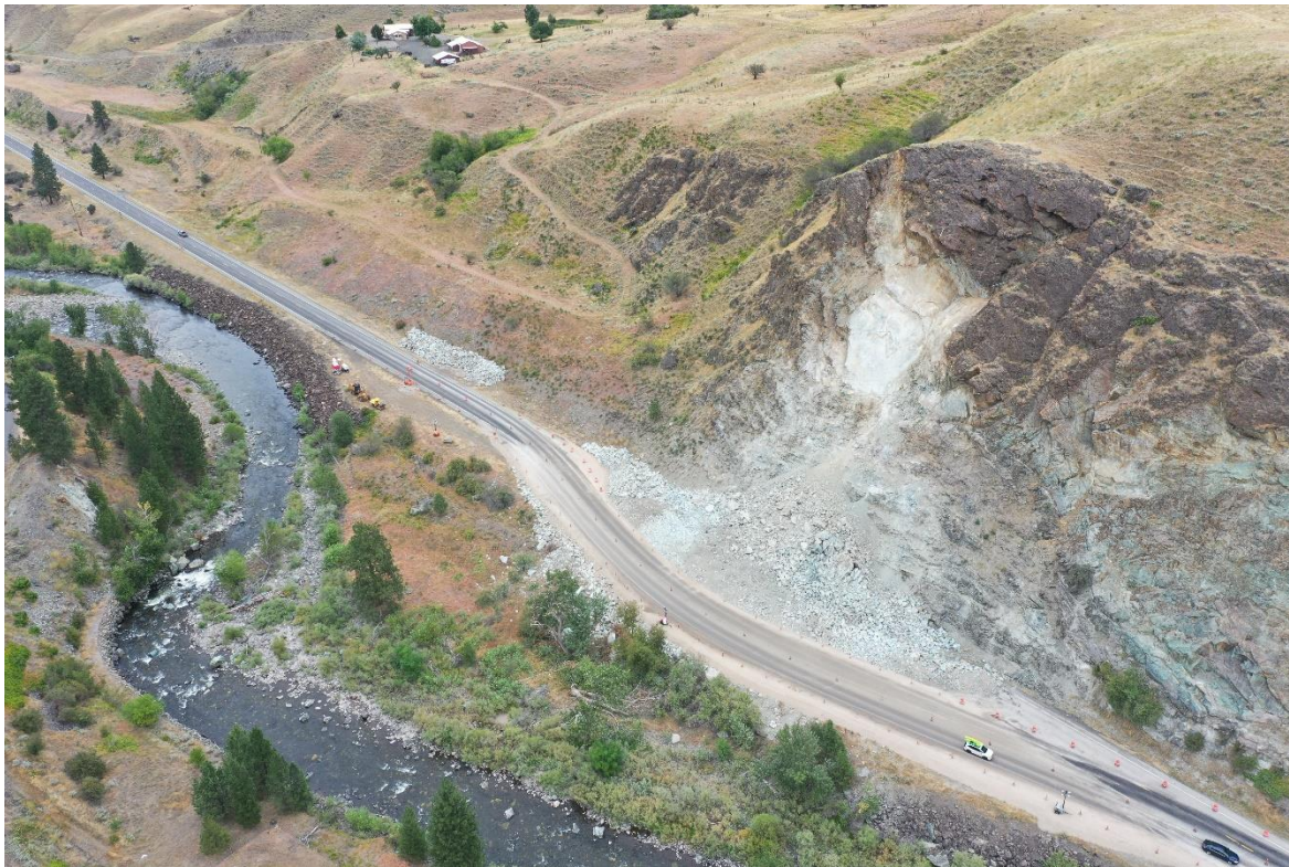
Figure 3.3 Oblique aerial photograph of rockfall along US-95 south of Riggins (45.331782°N, - 116.347058°E).
