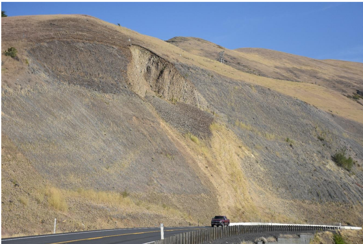
Figure 3.7 Photograph of a landslide in a basalt roadcut along SH-3 south of Juliaetta (46.482196°N, - 116.770068°E).
