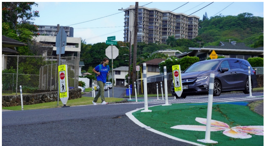
Figure 2: Supported by the Honolulu Complete Streets and Safe Routes to School Programs, Blue Zones Project Hawai'i partnered with the Stevenson Middle School leadership class to design and construct low-cost decorative curb extensions to enhance pedestrian safety by shortening the crosswalk distance, reduce illegal left turns out of the school's driveway, and slow the speed of vehicles. Blue Zones Project Hawai'i is a community-led initiative to improve health and wellness. (Image courtesy of City and County of Honolulu Department of Transportation Services)
