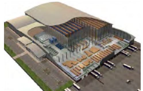
Fig. 20: Mega Warehouse and Cross Dock Source: GUS-EX
