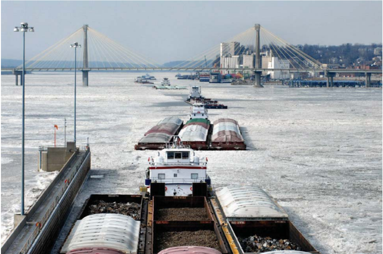
Figure 4.9: Tows delayed during ice conditions, Melvin Price Locks and Dam, Mississippi River, February 2007; ice build up in the lock caused one tow to become stuck, temporarily shutting down the lock; later, width restrictions were implemented (photo by Russell Elliott courtesy of US Army Corps of Engineers)
