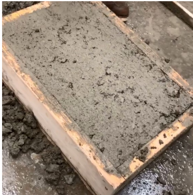
Figure A.15: Concrete finished surface after screeding and troweling (Mixture 4)
