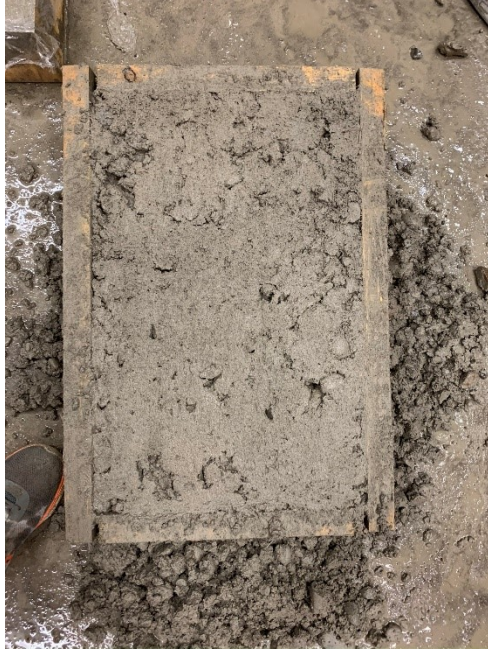
Figure A.38: Concrete finished surface after screeding and troweling (Mixture 11)
