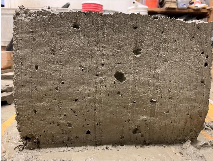
Figure A.57: Surface-void profile for one of the sides of box test specimen (Mixture 23)
