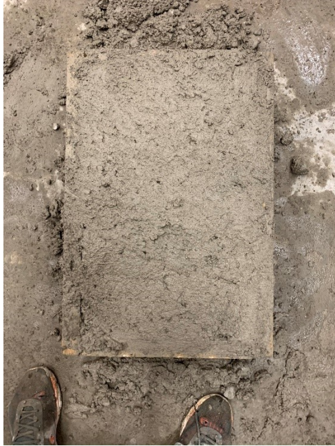
Figure A.59: Concrete finished surface after screeding and troweling (Mixture 23)
