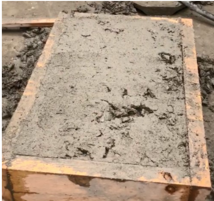
Figure A.11: Concrete finished surface after screeding and troweling (Mixture 3)
