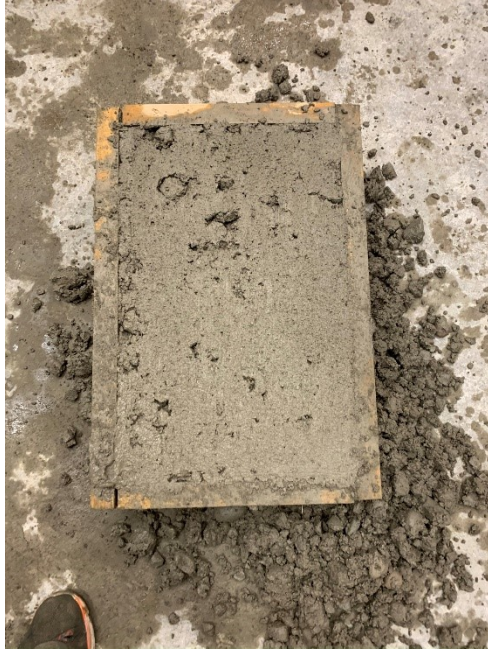
Figure A.56: Concrete finished surface after screeding and troweling (Mixture 22)
