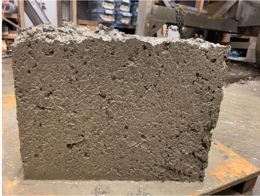
Figure A.20: Surface-void profile for one of the sides of box test specimen (Mixture 6)
