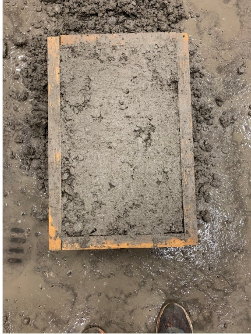
Figure A.46: Concrete finished surface after screeding and troweling (Mixture 14)
