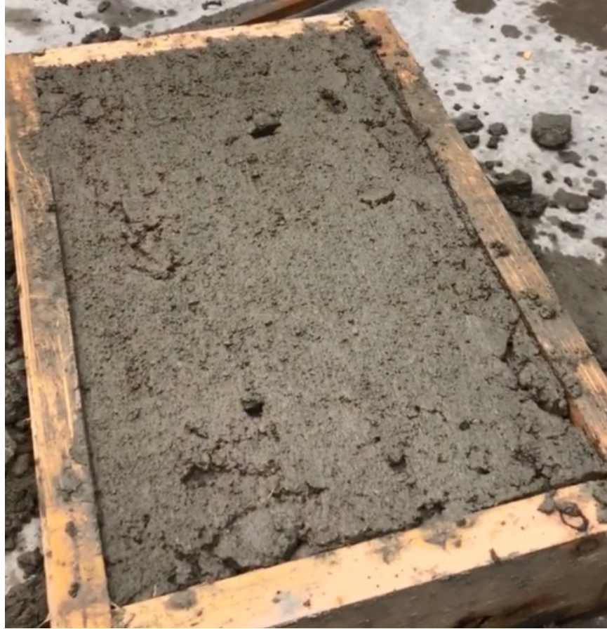
Figure A.7: Concrete finished surface after screeding and troweling (Mixture 2)
