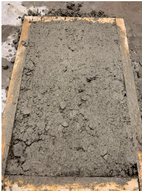
Figure A.19: Concrete finished surface after screeding and troweling (Mixture 5)
