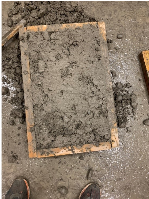
Figure A.52: Concrete finished surface after screeding and troweling (Mixture 16)
