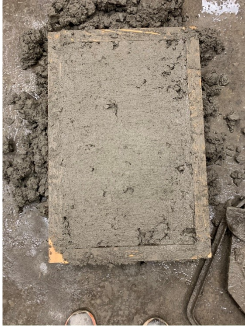
Figure A.41: Concrete finished surface after screeding and troweling (Mixture 12)
