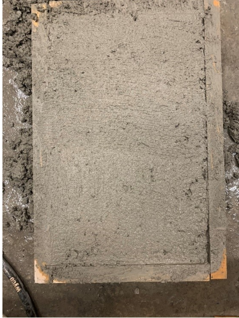
Figure A.50: Concrete finished surface after screeding and troweling (Mixture 15)
