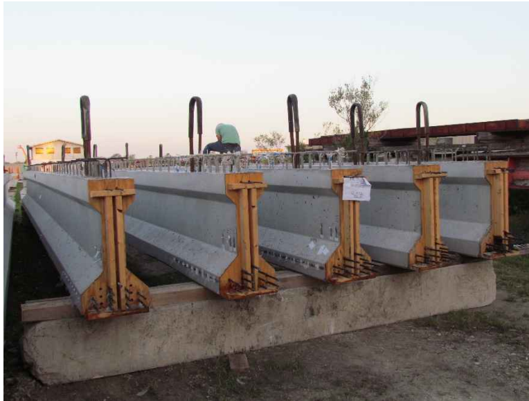
Figure 17 Girders at the casting yard
