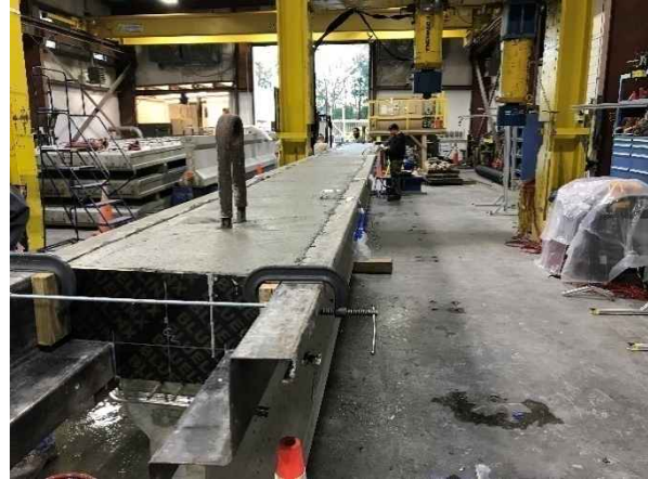
Figure 4-20 Girder after casting deck slab
