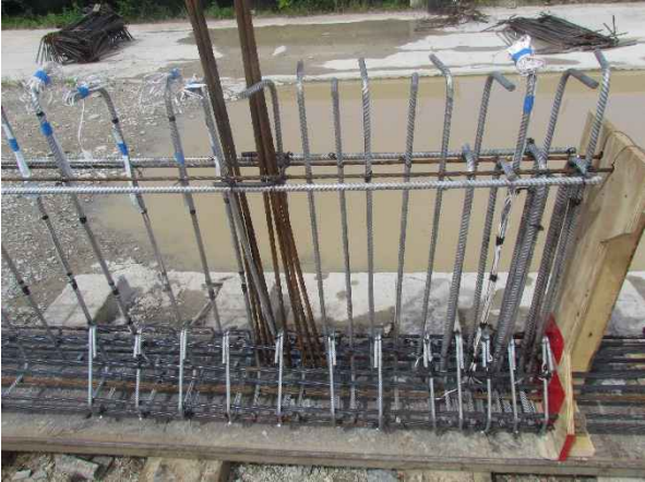
Figure 4-7 Stainless steel confinement reinforcement
