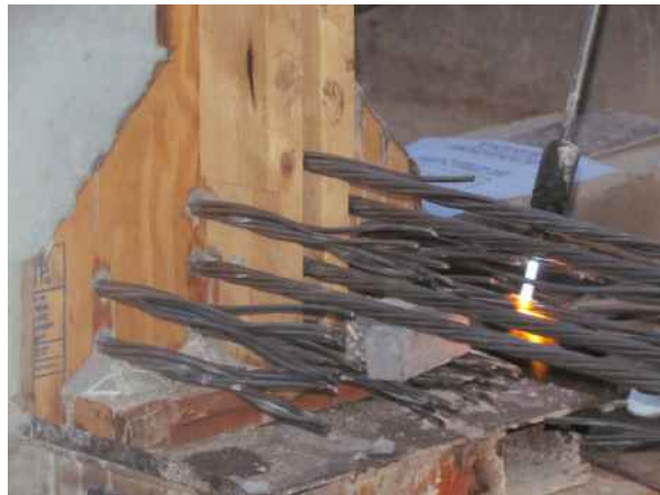
Figure 4-15 Releasing stainless steel strands using flame
