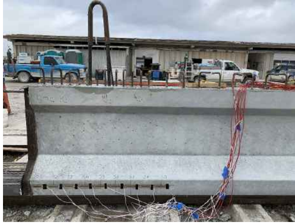
Figure 5-13 Installation of strain gages for transfer length
