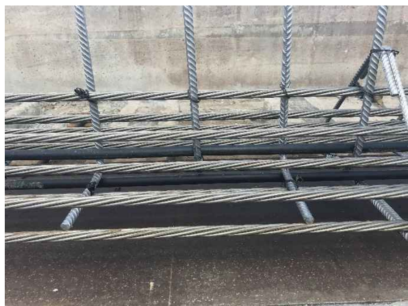
Figure 4-6 Shielding two strands in Girder B2
