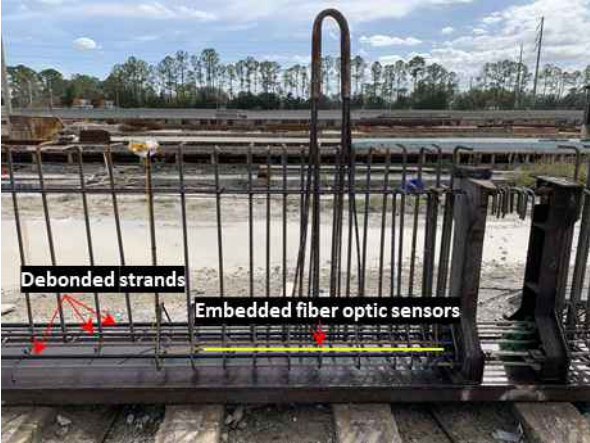
Figure 5-11 Installation of internal Fiber Optic Sensors for transfer length
