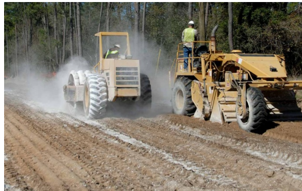
Figure 1. Chemically modified subgrade (courtesy Mintek Resources)
