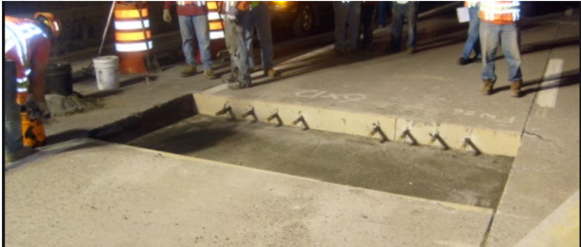
Figure 1. Full Depth Concrete Patch
