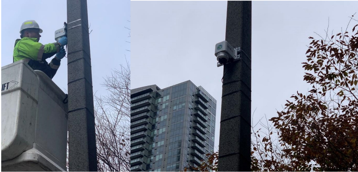
Figure 5-7 MUST Sensor Installed in Bellevue Test Bed
