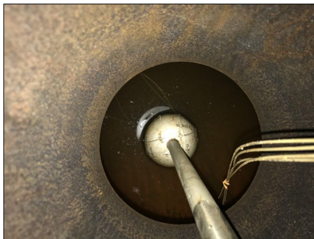
Figure 8. Float installed in tank, looking down through top nozzle
